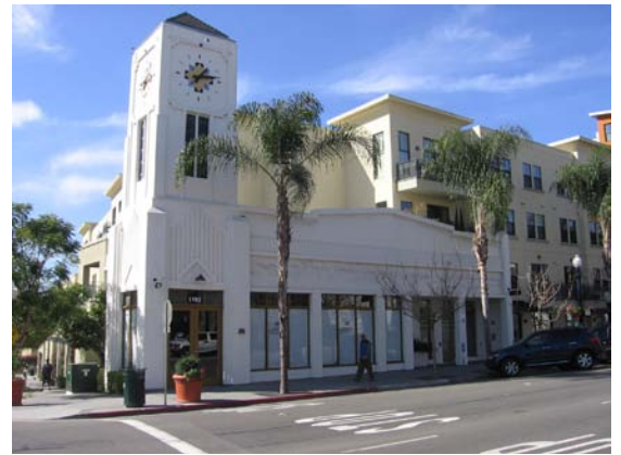
New residential development that wraps around an existing historic building, using building setbacks and a similar palette of materials and colors so as not to “overwhelm” the historic building
