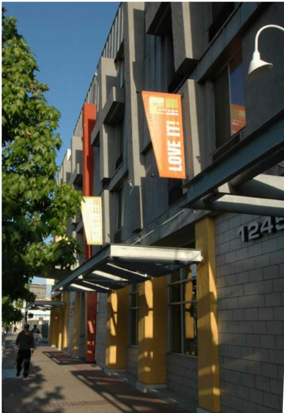
Awnings, canopies and overhangs, as well as a change in materials at the ground level, help to distinguish commercial from residential uses
