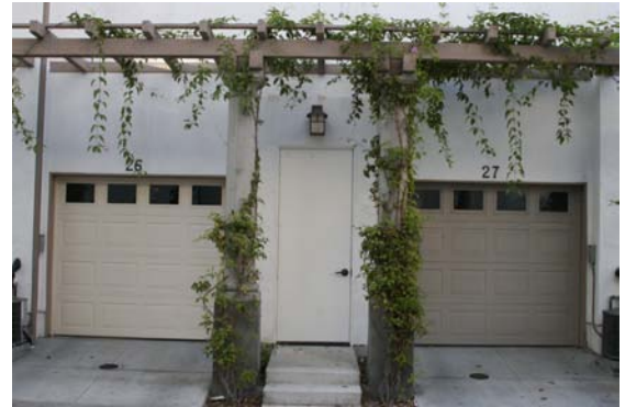
Carports and garages with shade structures and landscaping
