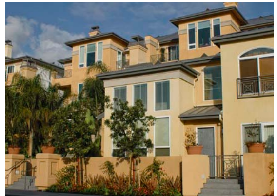
Varied building heights and upper floor setbacks provide an opportunity for different roof pitches and styles
