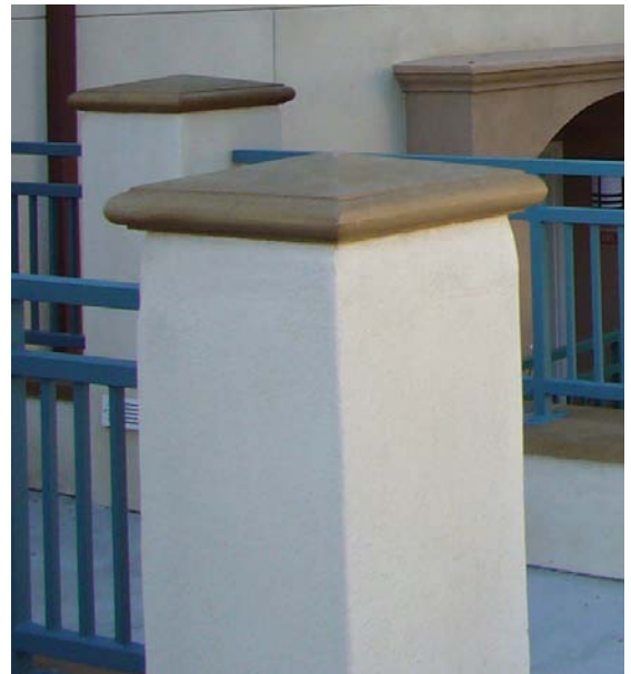
Capstones on pilasters, garden walls, and ledges can help minimize water damage and vandalism
