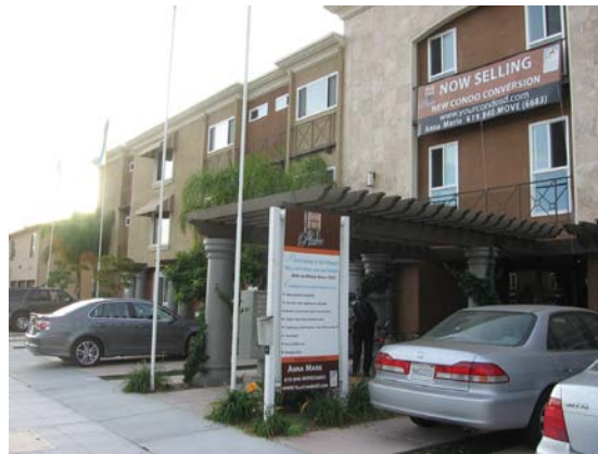
Design elements (such as awnings, railing, color and entry features) help make condominium conversions more appealing and provide a better street presence
