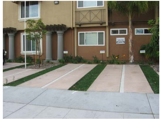
When parking cannot be relocated to the rear of the site, planting strips between parking stalls ("Hollywood Strips") are a good solution to softening parking in the front yard
