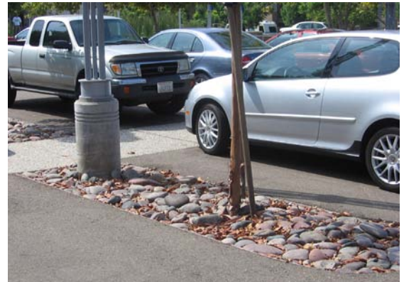
Provide opportunities for natural drainage and clearly marked pedestrian paths in parking lots
