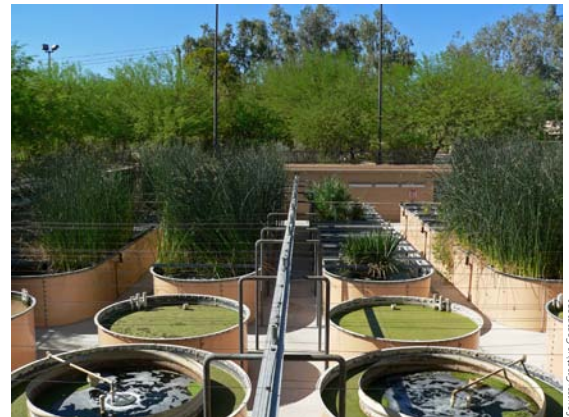
Greywater Tanks or "Living Machines" are one way to recycle and treat wastewater on-site
