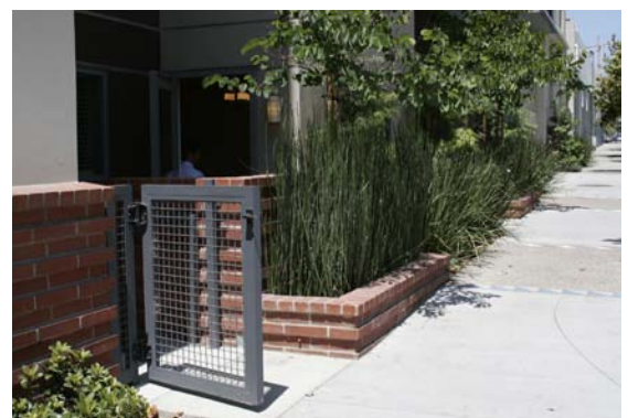
Individual dwelling unit gates and patio walls
