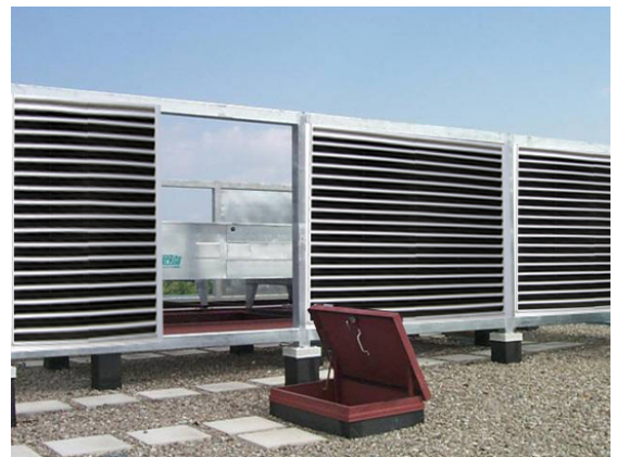
Heavy mechanical equipment that is normally located on the roof of a building should be enclosed with louvers, metal grates, or other screening materials to soften their visual impact on neighbors
