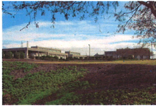
North City Water Reclamation Plant
