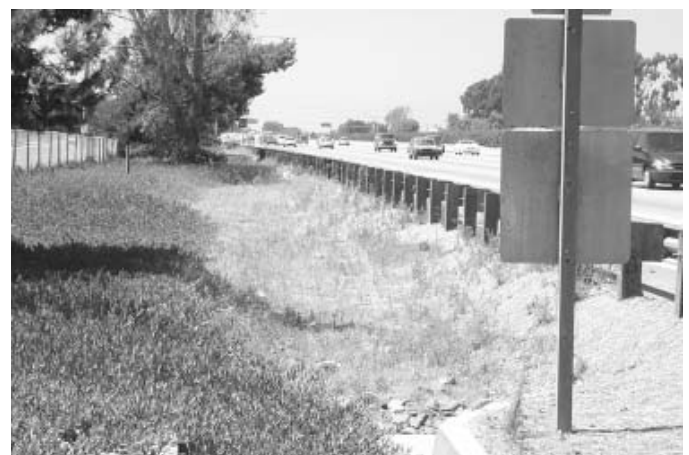
Figure 4 Vegetative Swale – Southbound Interstate 5 near La Costa Avenue Offramp
