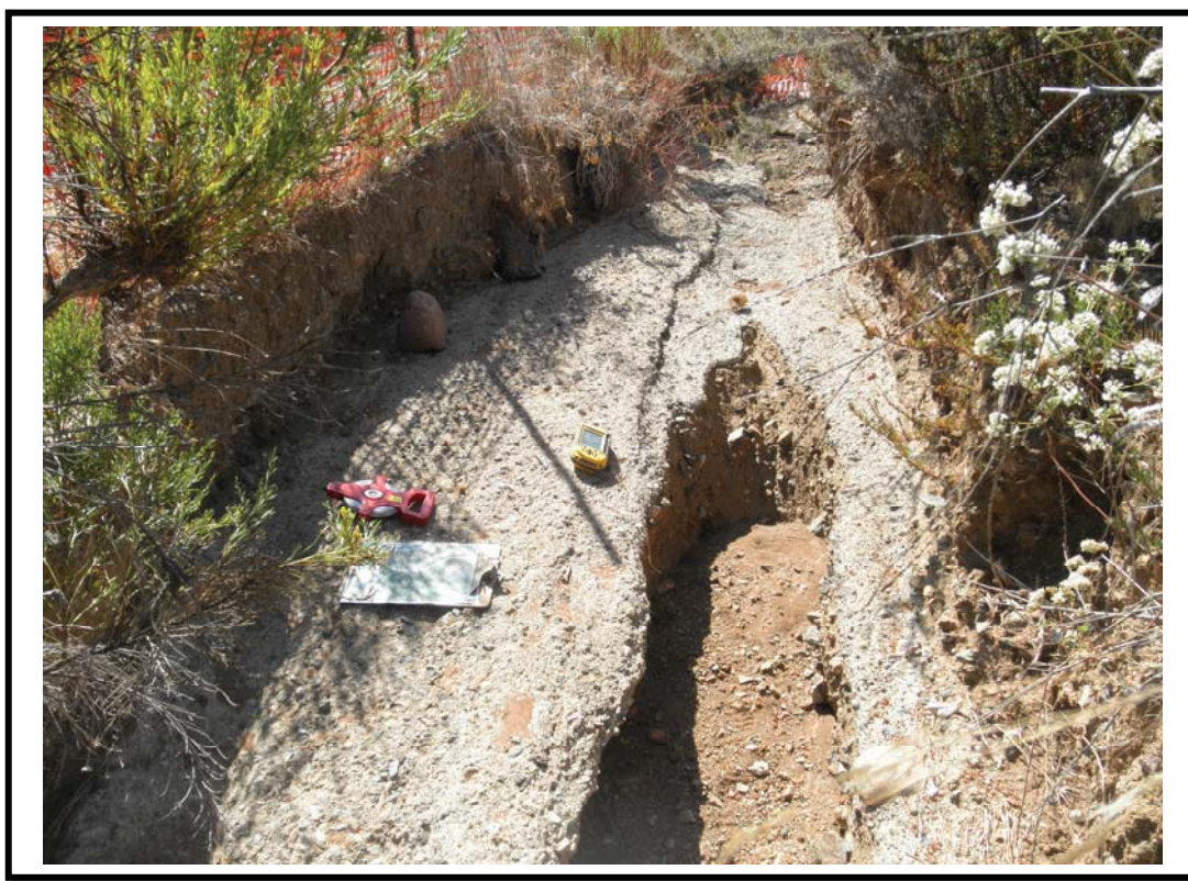
Photo Point 4. Headcut in channel adjacent to west side of Black Mountain access road.
