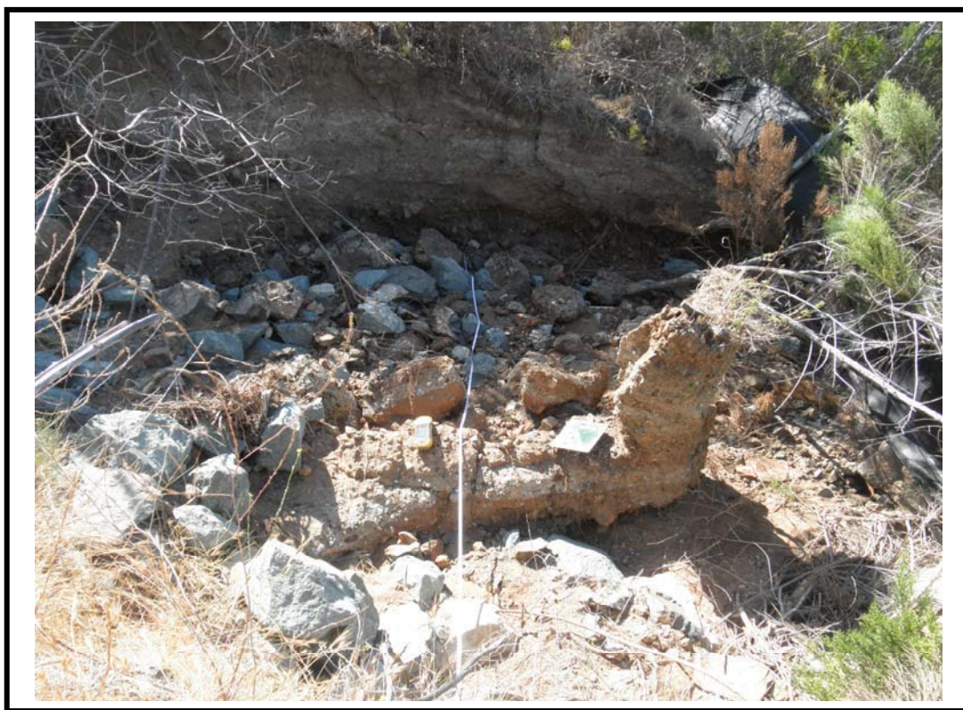
Photo Point 7. Extensive erosion at mouth of channel.
