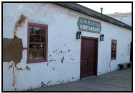
The Casa de Machado is an adobe house built in 1832 by Jose Manuel Machado as a wedding present for his daughter. The foundation is constructed of field stone laid in adobe mortar. The walls consist of sun dried adobe brick laid in adobe mortar, plastered on both sides with adobe mortar and white washed.
