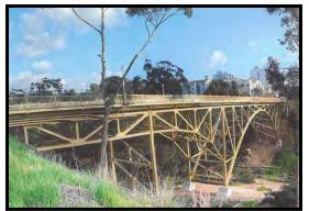
The First Avenue Bridge is significant in its engineering and architectural design as the only metal truss bridge in the City of San Diego and one of a handful of arch truss bridges located in the State of California. Completed in 1931, the First Avenue Bridge over Maple Canyon is among the most visible and important manifestations of early 20<sup>th</sup> century civil engineering
