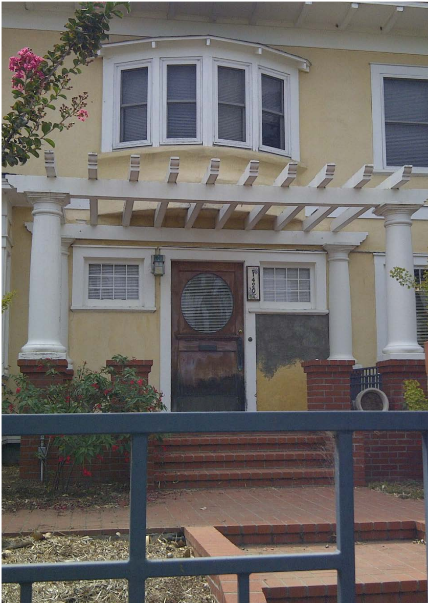
Front Door in 2013 Prior to Unpermitted Alteration
