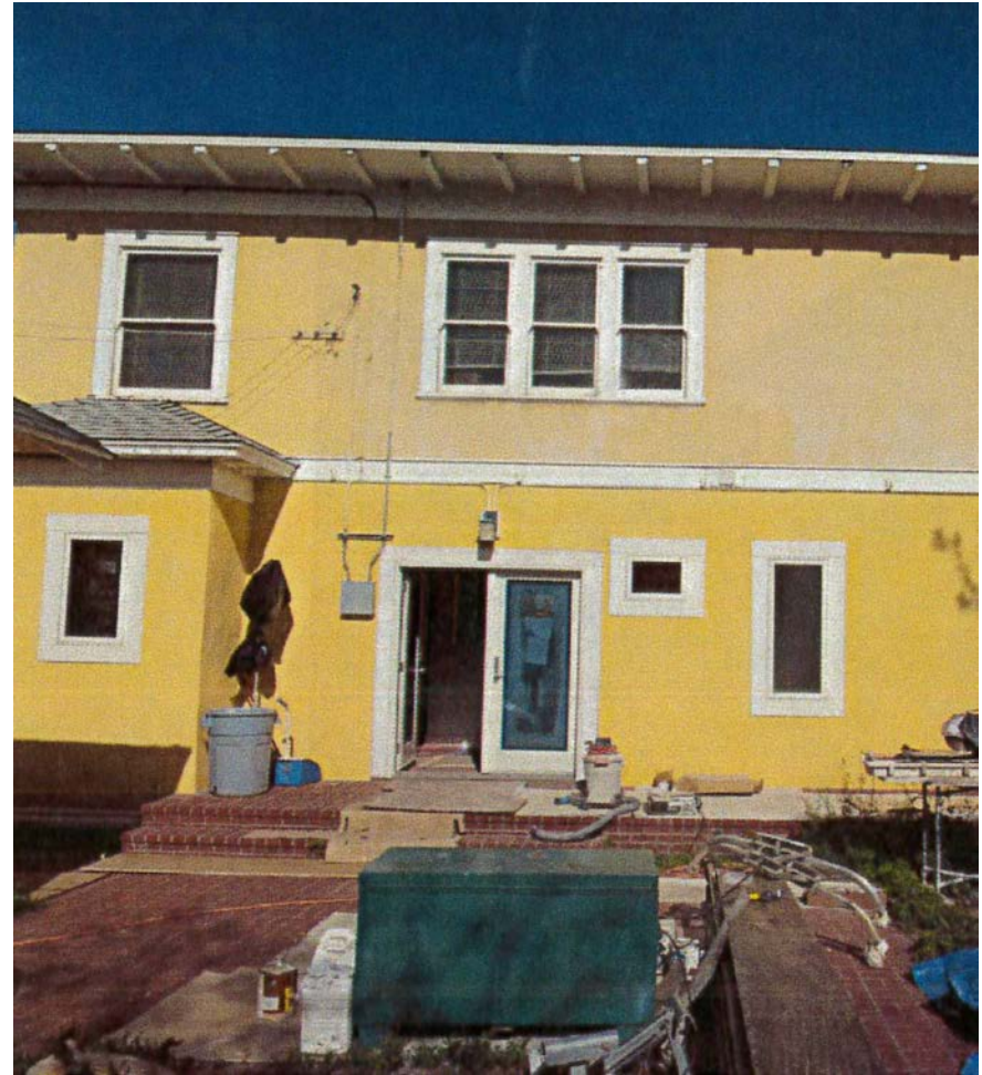
Rear After Unpermitted Alteration
