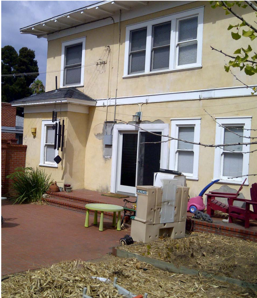
Rear in 2013 Prior to Unpermitted Alteration
