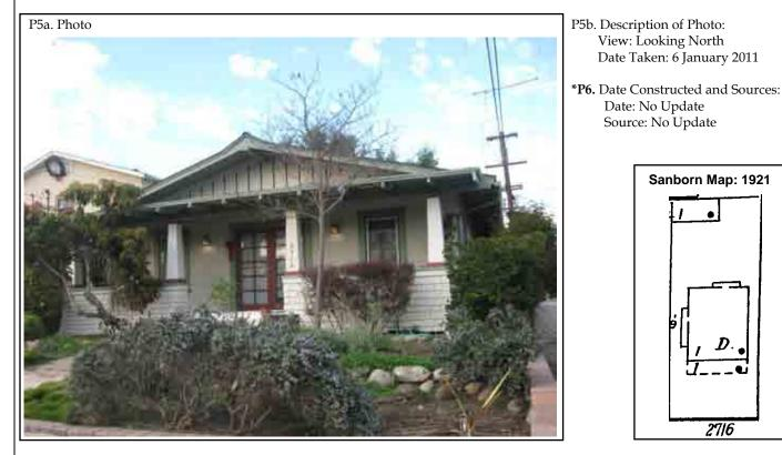
\*B6. Construction History: (Construction date, alterations, and date of alterations) Vinyl windows have been installed along the east alley elevation within the original window openings, and one vinyl window has replaced the original wood frame and sash window in the original opening on the front elevation. The original scored concrete walkway has been removed and replaced with pavers, and a low retaining wall has been constructed at the front and side property lines.
