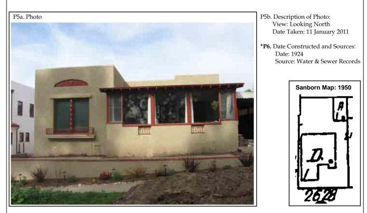
\*B6. Construction History: (Construction date, alterations, and date of alterations) A large addition was constructed at the front of the house. A thicker, historically inappropriate stucco texture has been applied to the house. A metal carport has been added at the east side of the house. A low retaining wall has been constructed at the front yard.
