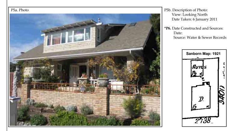
\*B6. Construction History: (Construction date, alterations, and date of alterations) The siding at the ground floor is a composition siding that has been installed over the original lap siding intact underneath. The original second floor sleeping porch/dormer was extended forward at some point. The original stepped walkway has been removed; the yard leveled; and enclosed with a brick wall.
