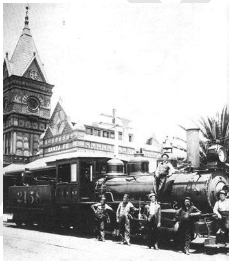
Figure 940: San Diego's Santa Fe Depot, 1887.
