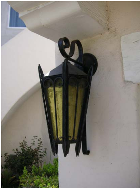
Photo 15: Corbel and original electric lamp on southwest elevation of garage.
