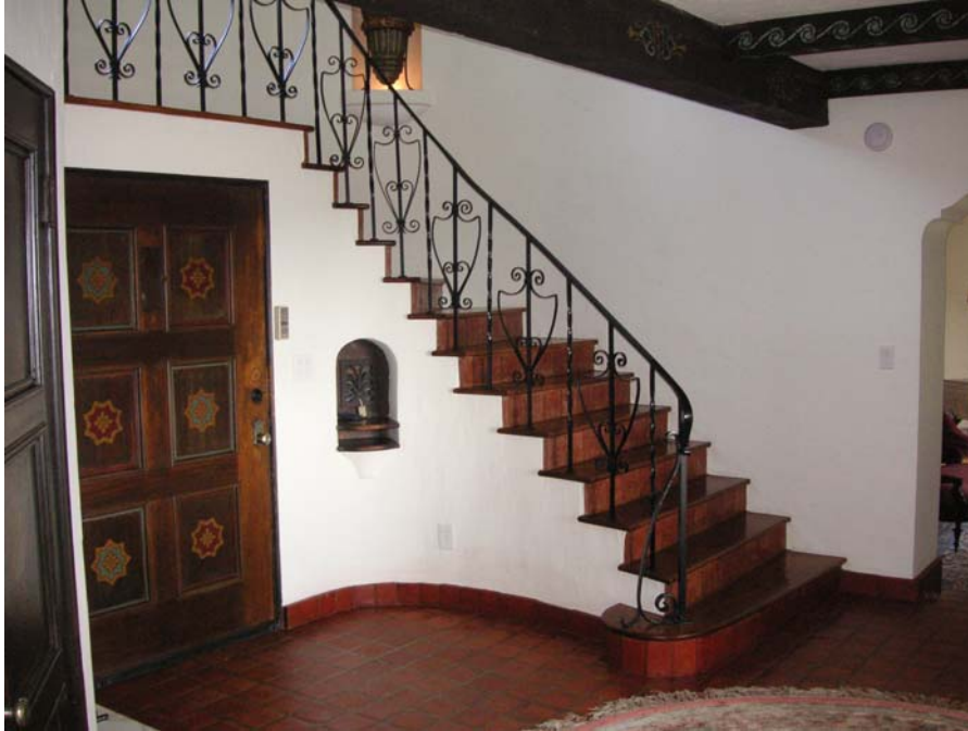
Photo 19: Stencil work on main entry door and decorative niche.
