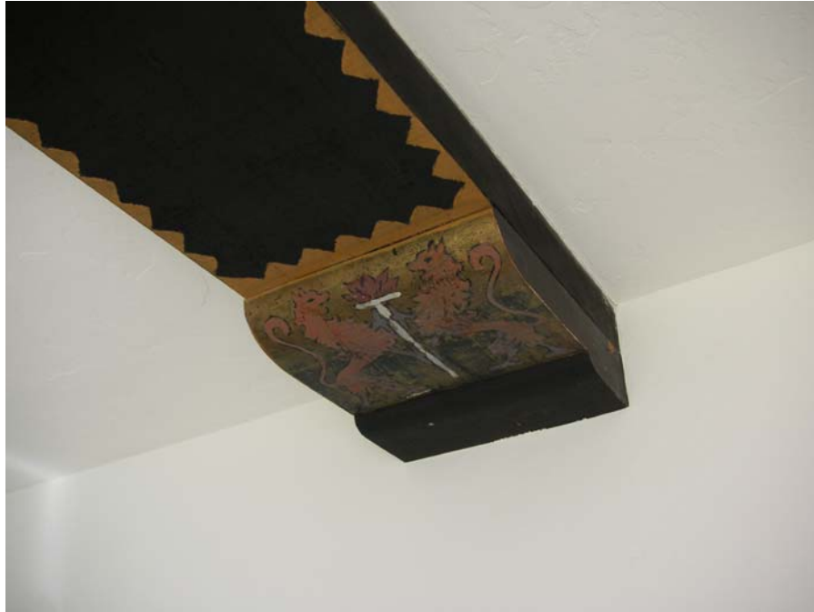
Photo 17: Stencil work on corbel and rafter in the Dining Room.
