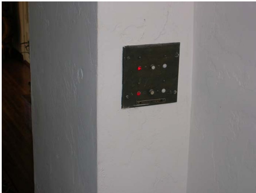
Photo 10: Original heat control and light switch panel.
