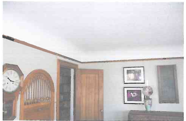
Photo 10: Coved ceilings: living room and dining room
