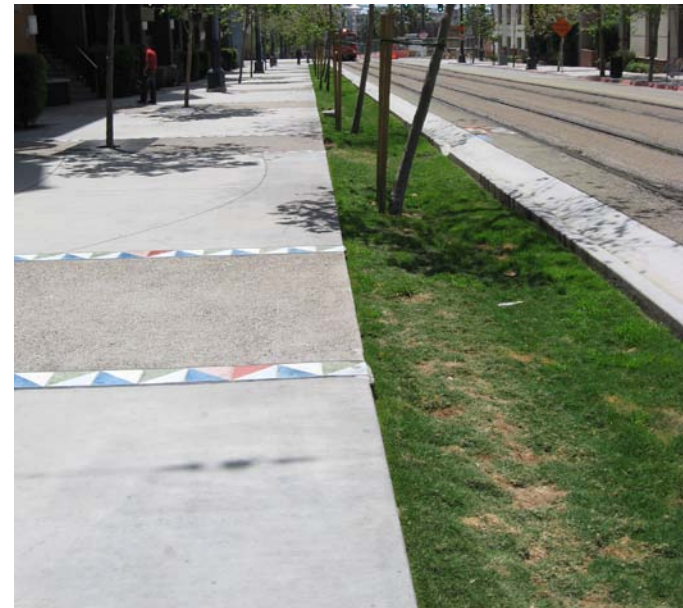
Example of an infiltration basin
