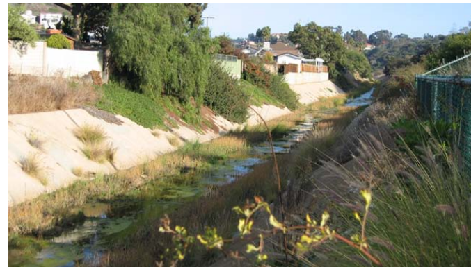
Hard surfaced channels such as Tecolote Creek increase velocity, prevent groundwater recharge and offer little wildlife habitat
