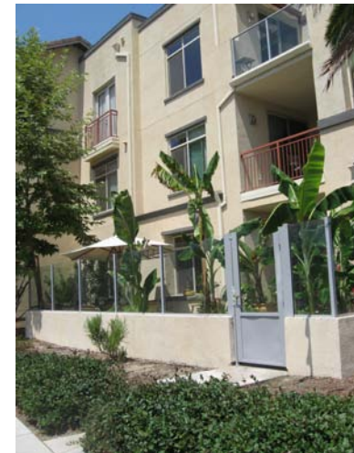
Example of outdoor patios and balconies adjacent to the River Corridor
