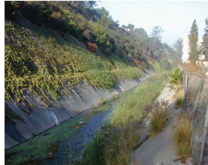
Vegetation can soften the impact of concrete channels
