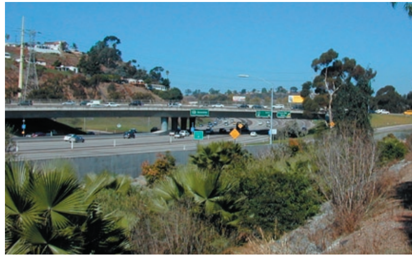
Murray Creek along SR-163
