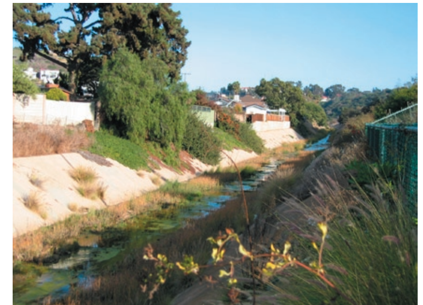
Channelization of Tecolote Creek
