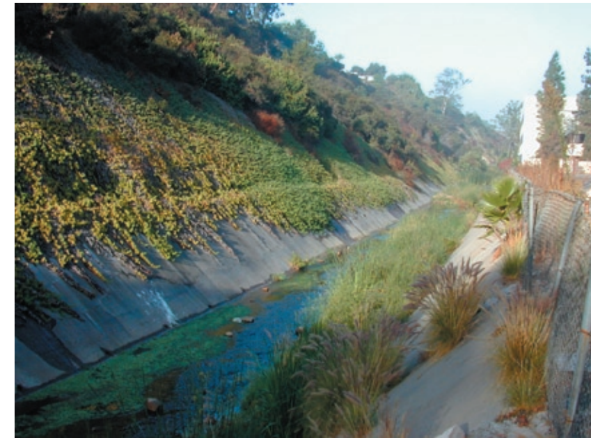
Channelized Alvarado Creek behind Medical Center
