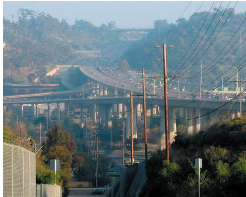
Highway infrastructure and rights-of-ways consume much of the valleys and canyons
