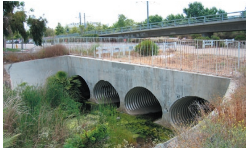
Culverts under alignment of Hazard Center Drive future extension
