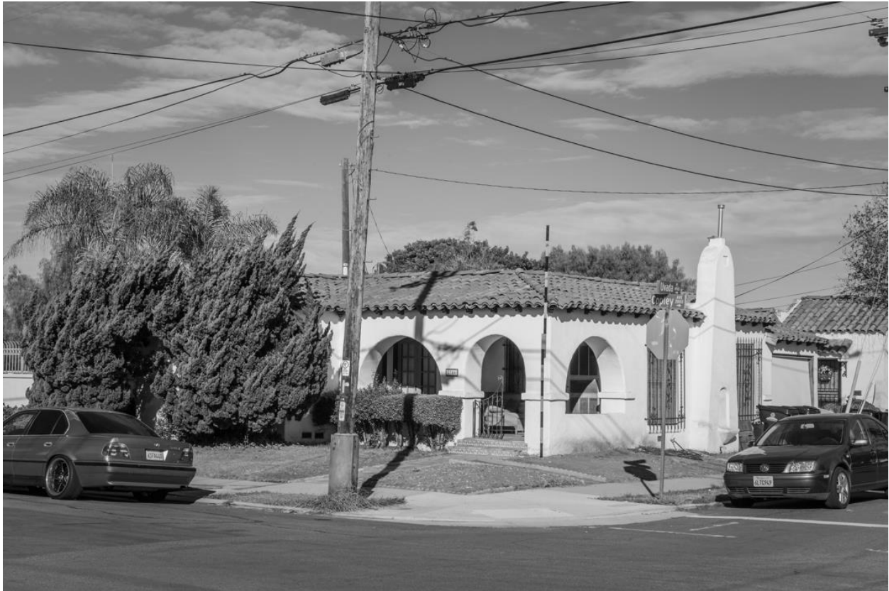
Figure 14: 2746 Copley, view northwest of property from the intersection of Copley Avenue and Uvada Place. Image Source: IS Architecture, December 2013.
