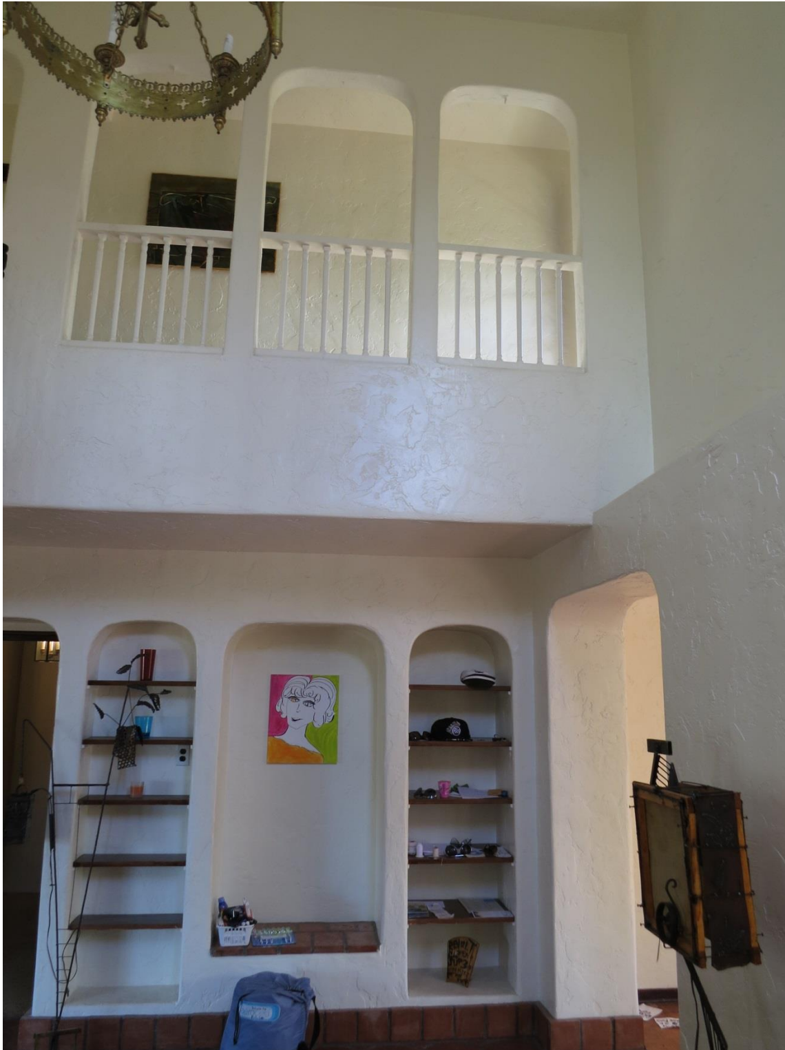
Figure 10: 2544 Collier, railing. Image Source: IS Architecture, December 2013.
