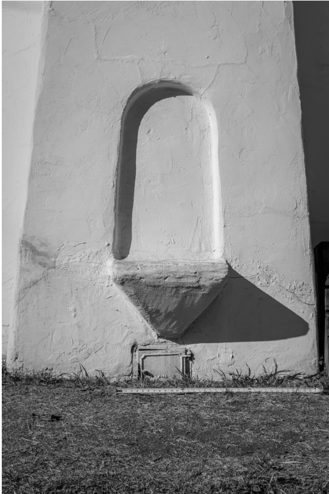
Figure 17: 2746 Copley, detail view of fireplace niche. Image Source: IS Architecture, December 2013.
