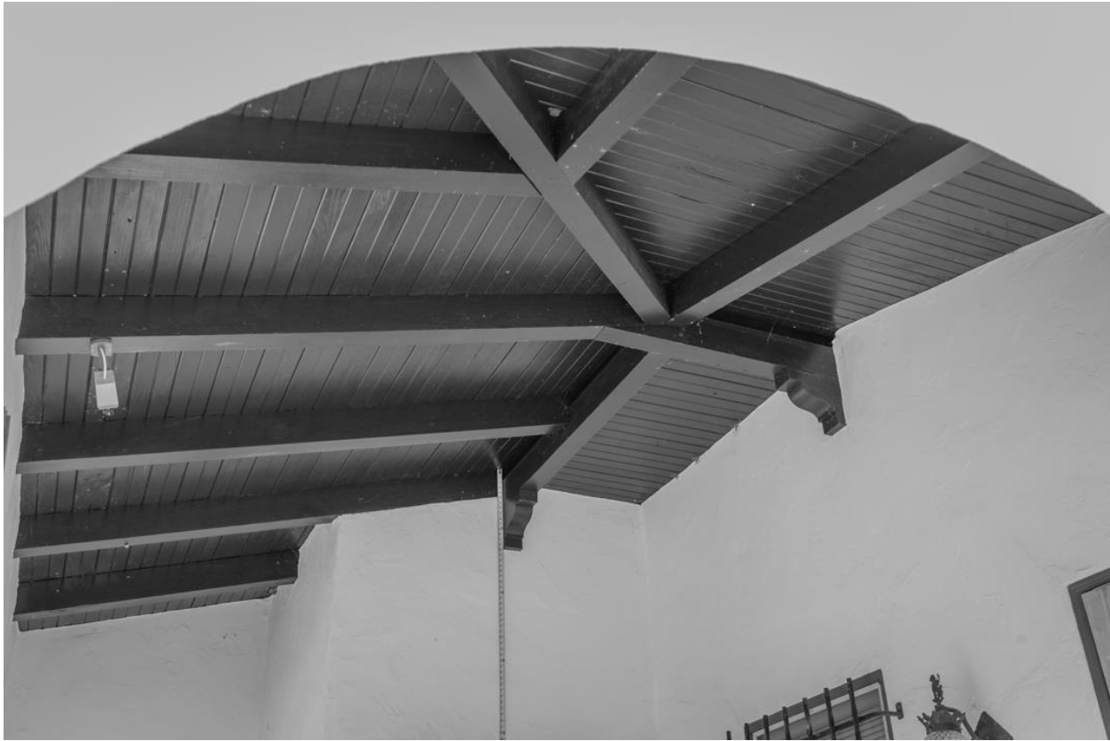
Figure 19: 2746 Copley, detail view of porch ceiling and roof framing. Image Source: IS Architecture, December 2013.
