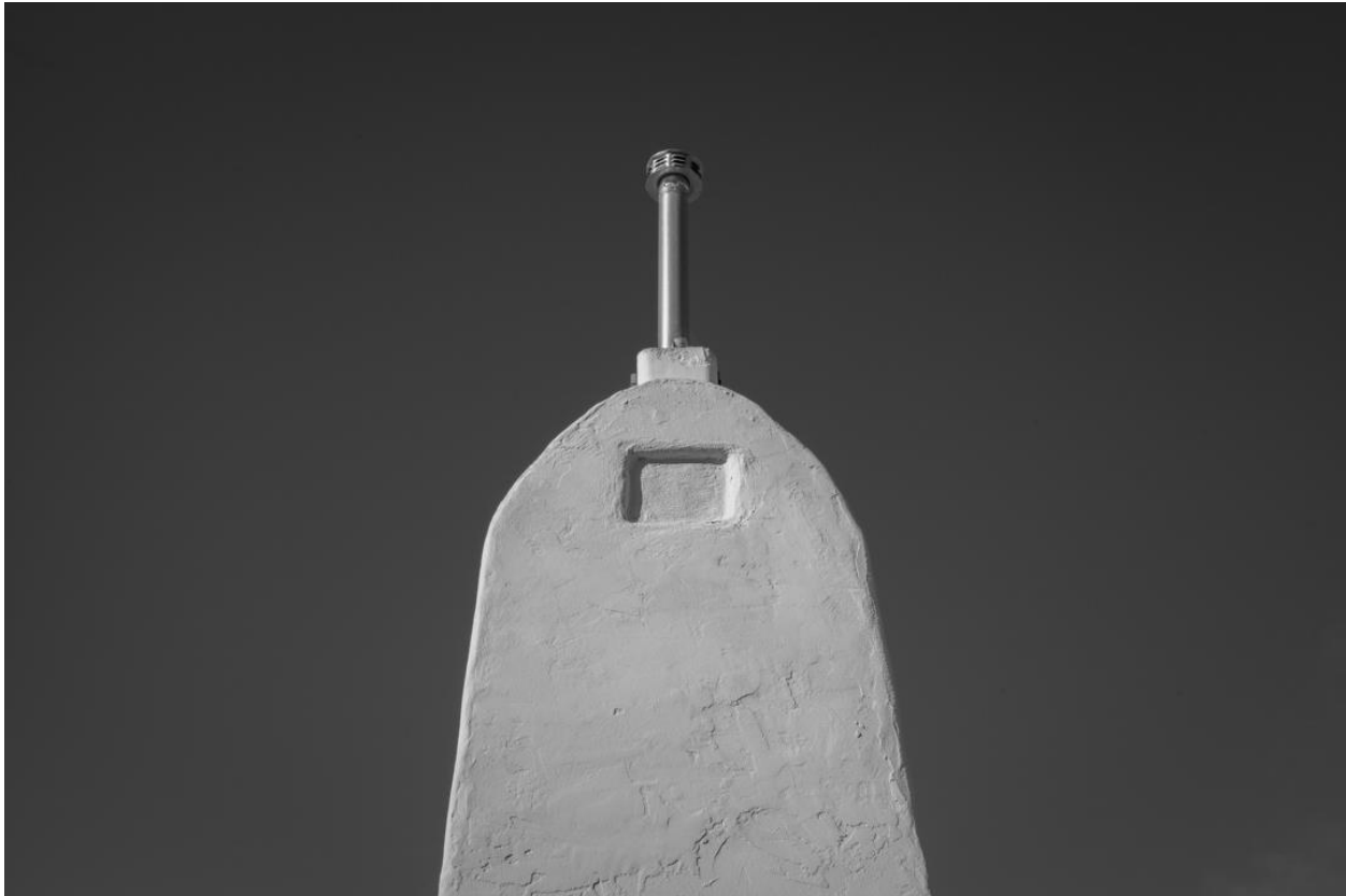
Figure 18: 2746 Copley, detail view of chimney. Image Source: IS Architecture, December 2013.
