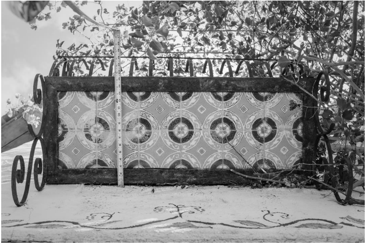
Figure 5: 2544 Collier, detail view of decorative scrolled iron balcony with tile base over front entry door. Image Source: IS Architecture, December 2013.
