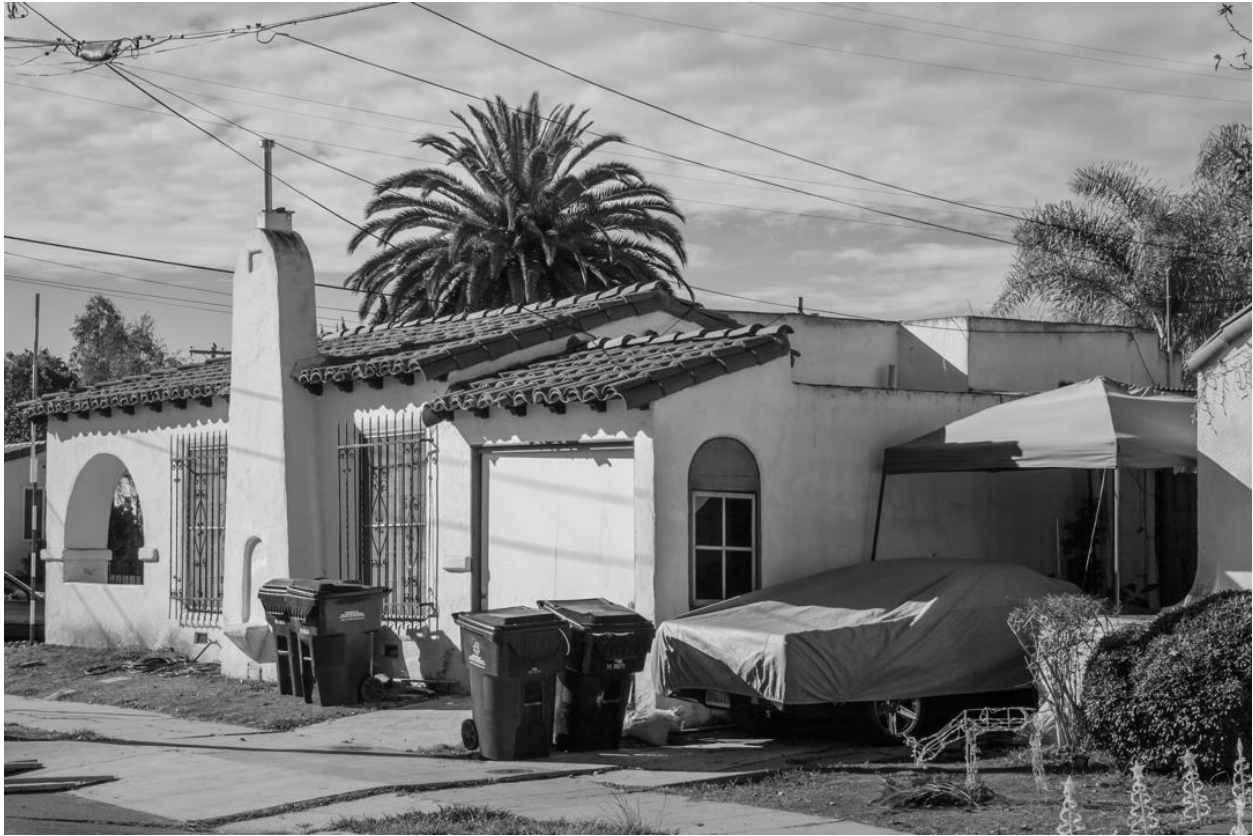
Figure 16: 2746 Copley, view southwest. Image Source: IS Architecture, December 2013.
