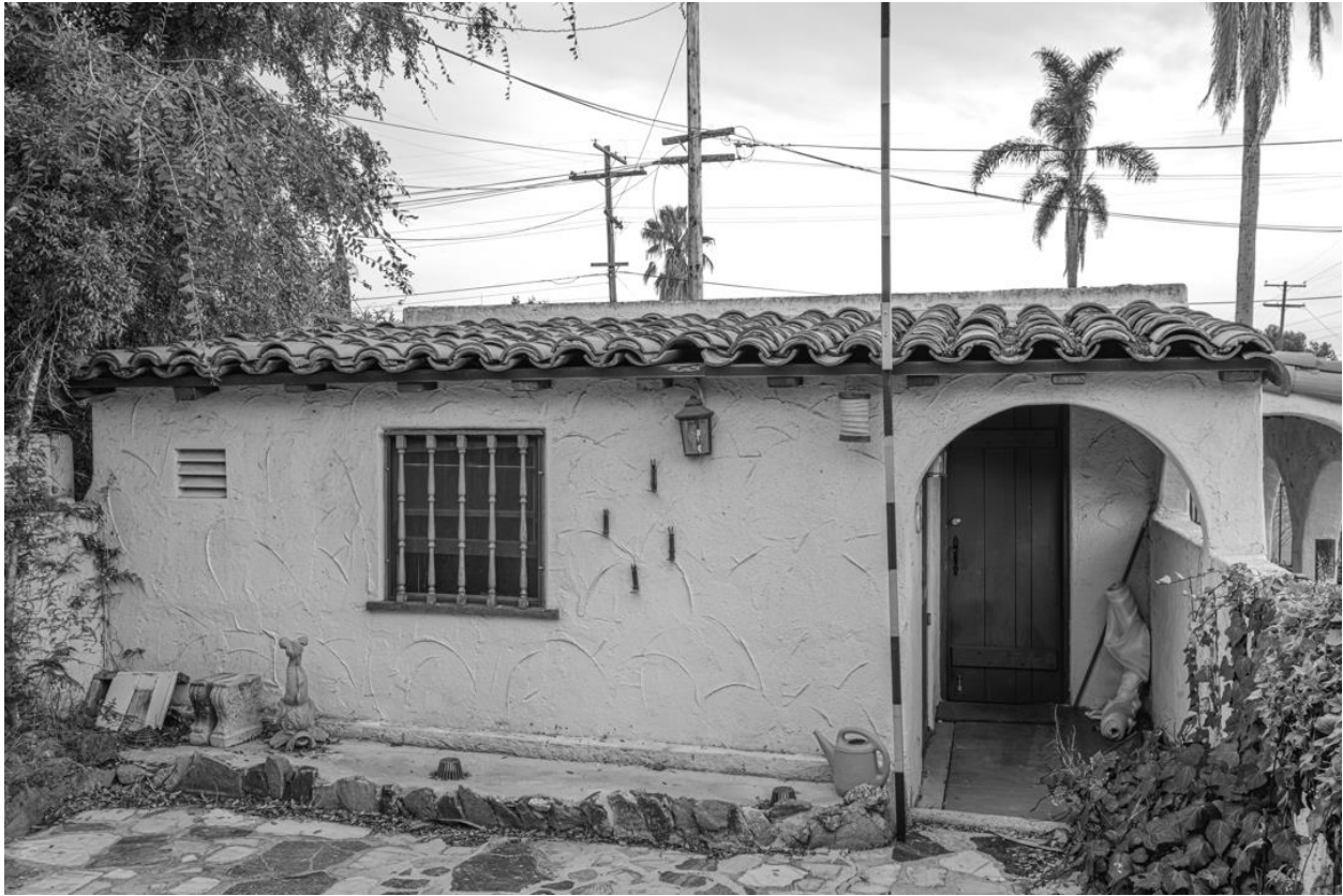
Figure 3: 2544 Collier, view south of north facade of garage. Image Source: IS Architecture, December 2013.
