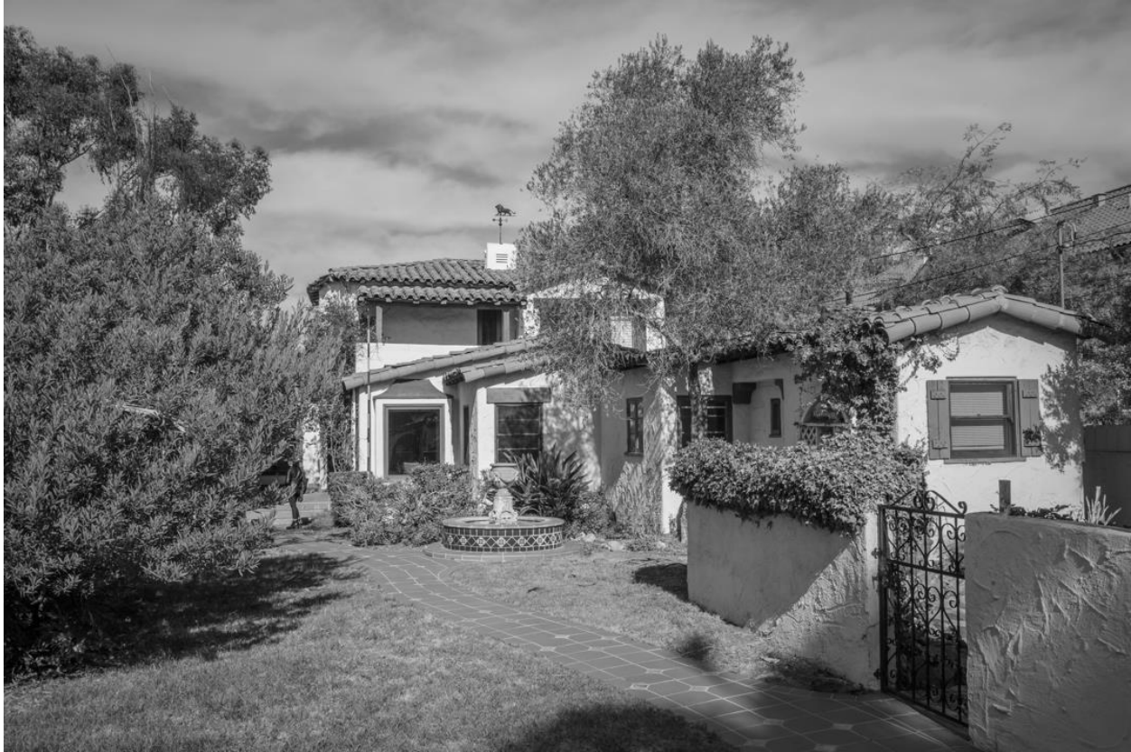
Figure 1: 2544 Collier, view north. Image Source: IS Architecture, December 2013.
