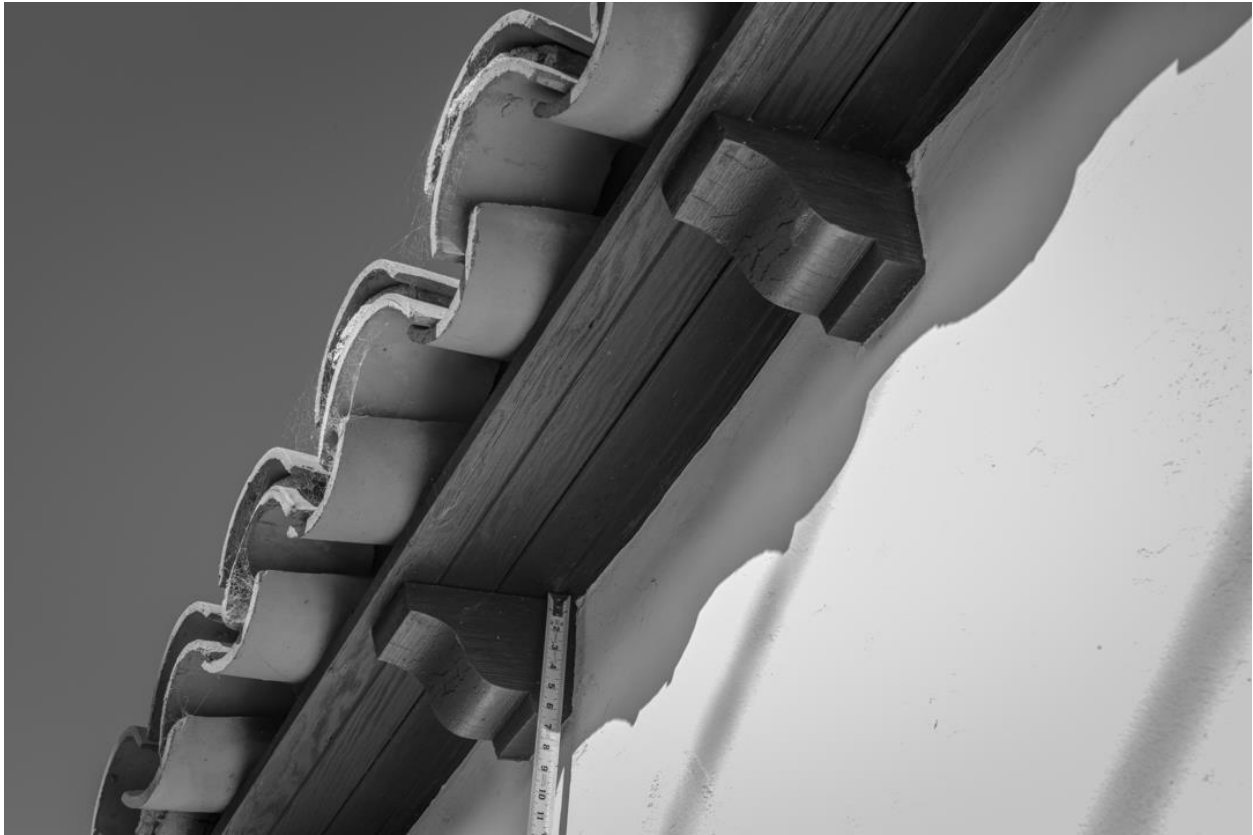
Figure 21: 2746 Copley, detail view of wood corbels showing vertical dimension. Image Source: IS Architecture, December 2013.
