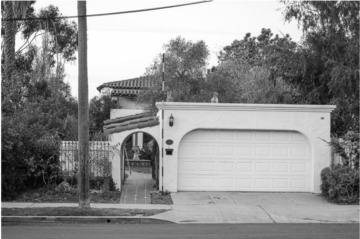
Figure 4: 2544 Collier, view north of property from Collier Avenue. Image Source: IS Architecture, December 2013.
