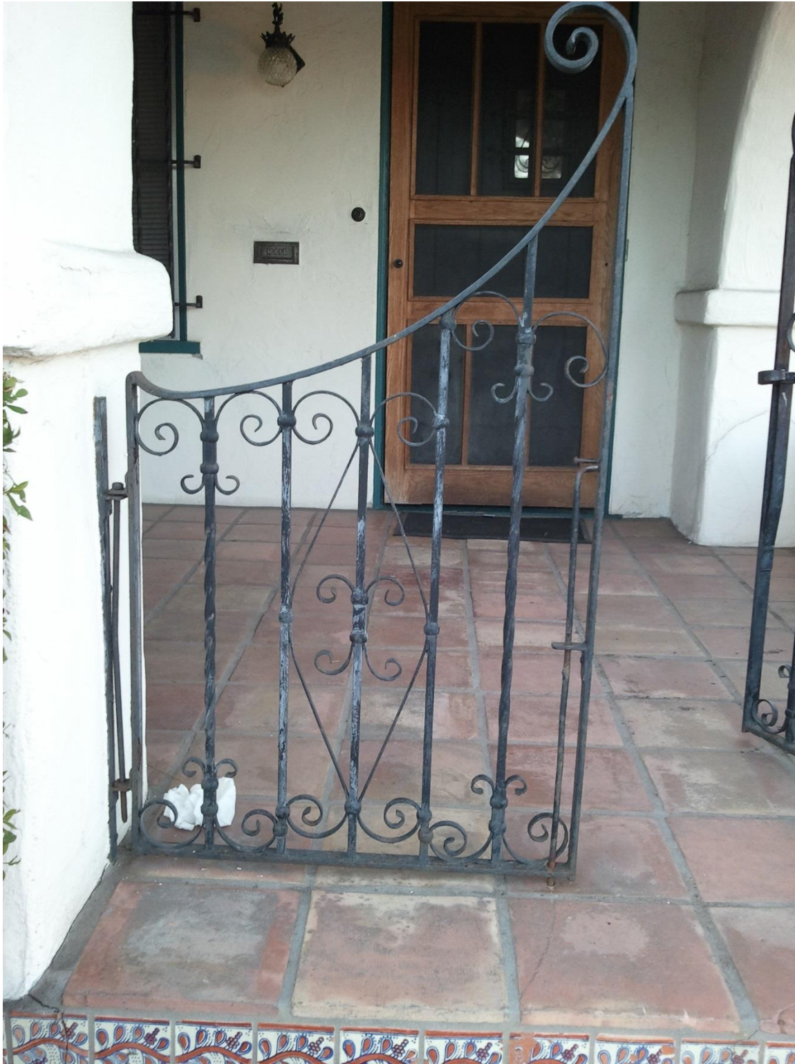
Figure 23: 2746 Copley, detail view of original Iron Gate. Image Source: IS Architecture, December 2013.
