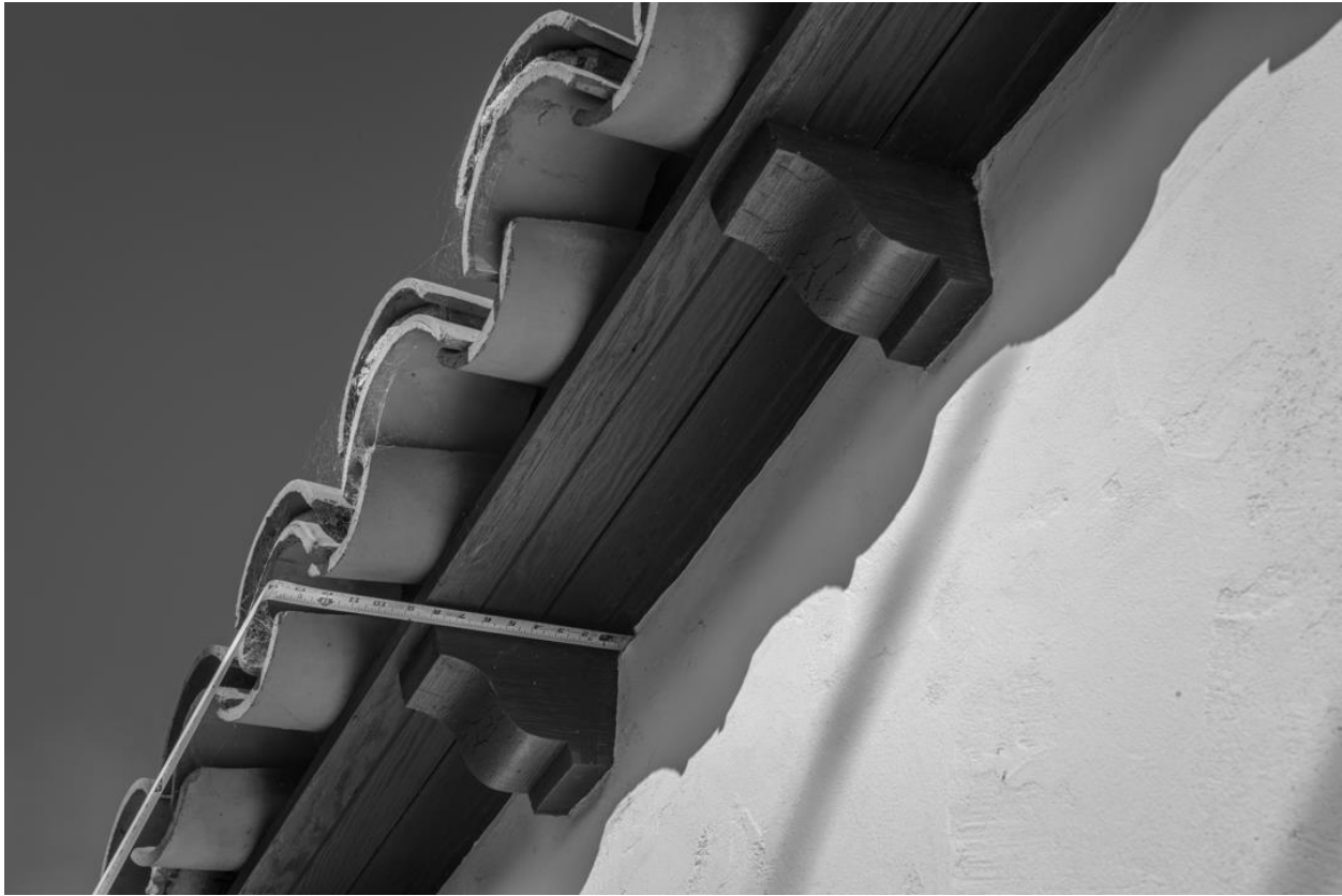
Figure 22: 2746 Copley, detail view of wood corbels showing horizontal dimension. Image Source: IS Architecture, December 2013.
