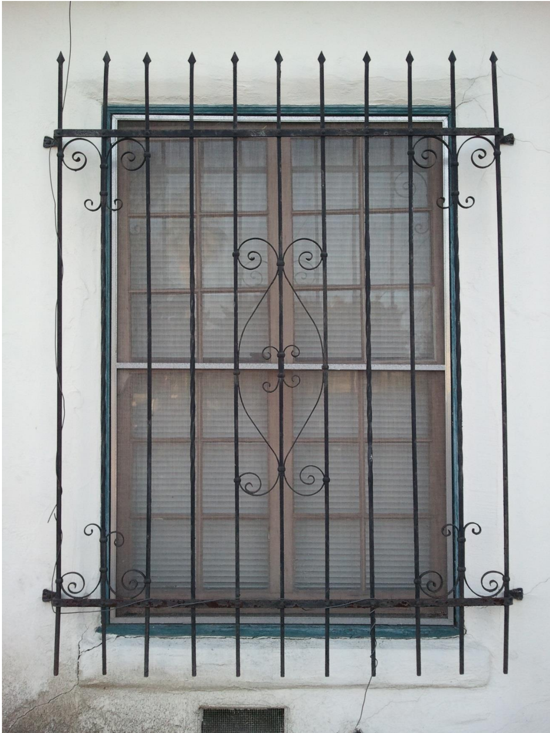
Figure 24: 2746 Copley, detail view of original Security Iron. Image Source: IS Architecture, December 2013
