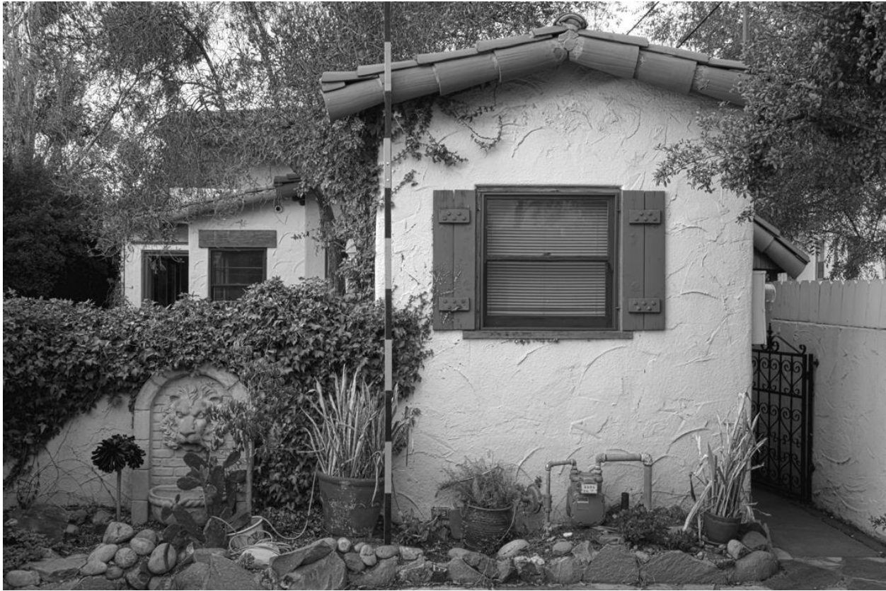
Figure 2: 2544 Collier, view north of most southern portion of house. Image Source: IS Architecture, December 2013.
