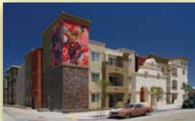
La Entrada Family Apartments Barrio Logan
