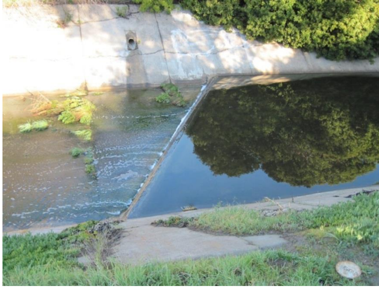
Figure K-17 Low-Flow Diversion in Tecolote Creek Subwatershed
