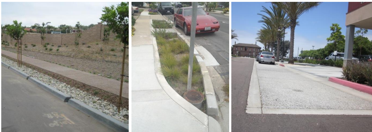
Figure 4-6 Examples of Bioretention and Permeable Pavement in the Right-of-Way with Curb and Gutter
