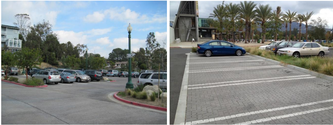
Figure 4-4 Permeable Pavement Functions as a Parking and Driving Surface While Capturing and Treating Storm Water
