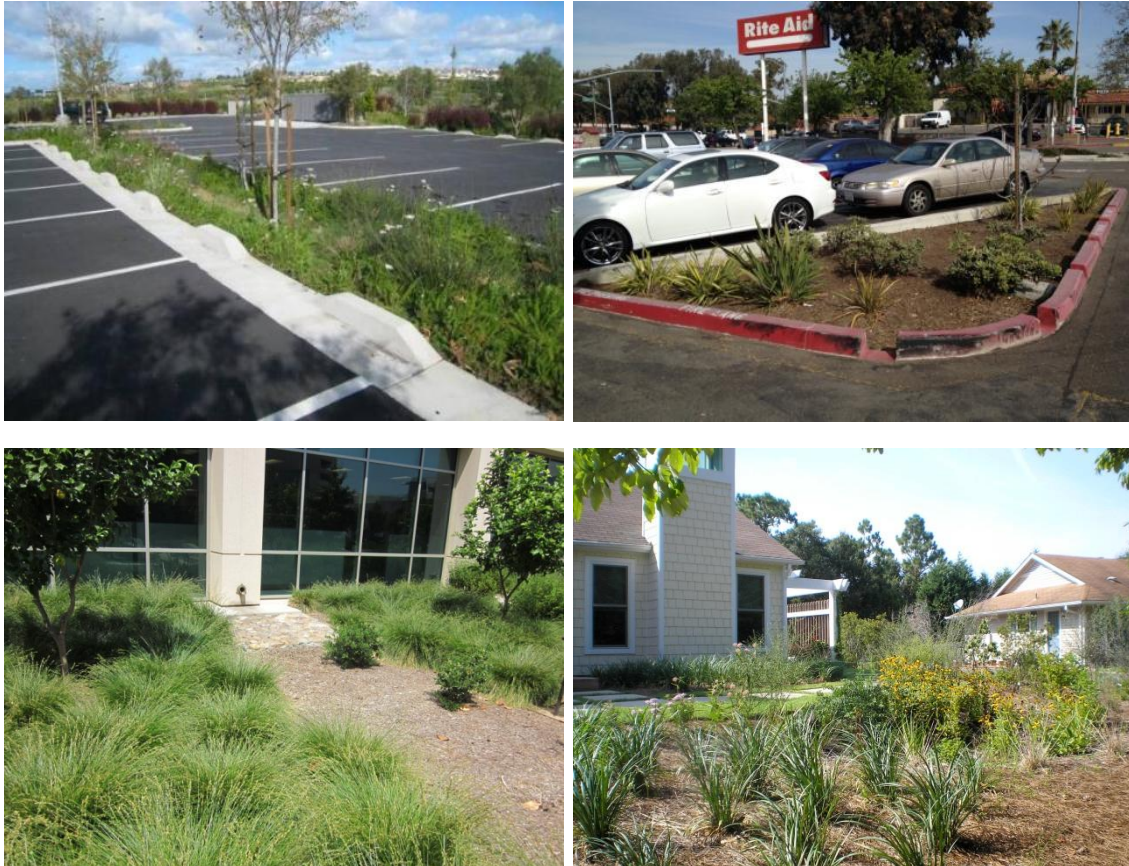
Figure 4-3 Bioretention Areas in Parking Lots and Adjacent to Buildings Provide Multiple Benefits by Treating Runoff While Also Serving as Landscape Features and Habitat
