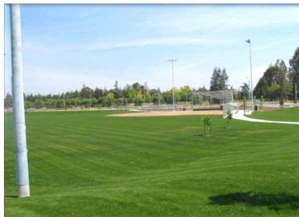
Figure 4-8 Example of an Athletic Field Designed to Function as an Infiltration Basin
