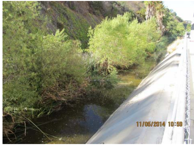
PHOTO NOTES: Reach Upper 2, looking downstream from the upstream end.
