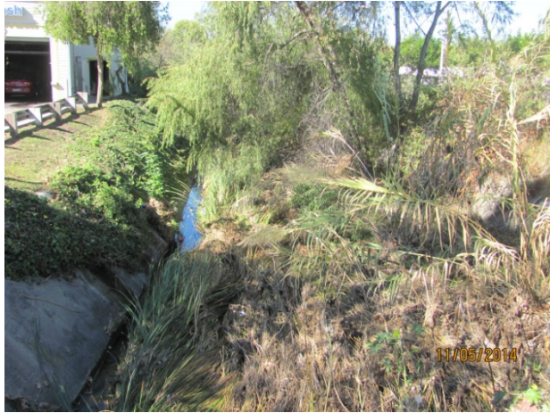
PHOTO NOTES: Reach Lower 2A, looking downstream from Fairmount Avenue.
