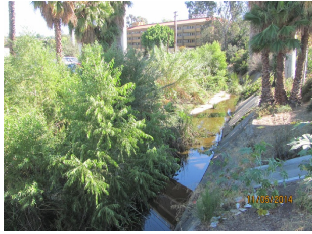
PHOTO NOTES: Reach Lower 2B, looking upstream from Fairmount Avenue.
