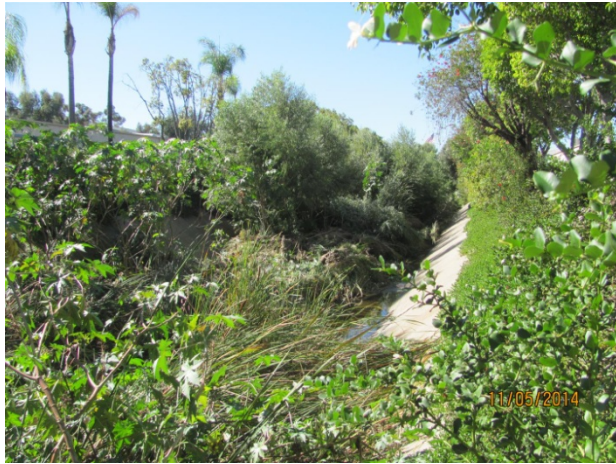
PHOTO NOTES: Reach Lower 2B, looking downstream from the upstream end.
