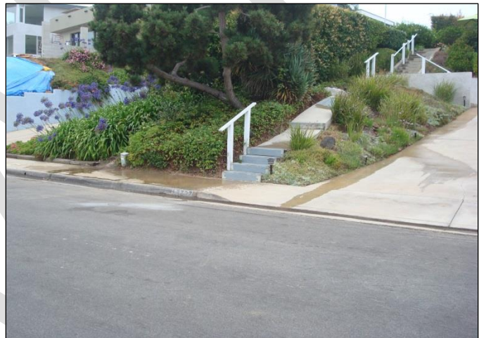
Evidence of irrigation runoff from over-watering/overspray on residential properties
