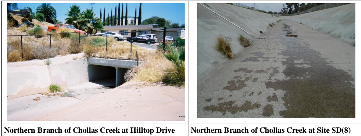
Figure 1-5. Channelization of the Chollas Creek Watershed
