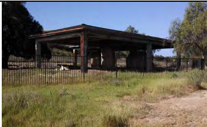
View NE: The Ruiz-Alvarado Adobe with a perimeter fence and protective roofing.
