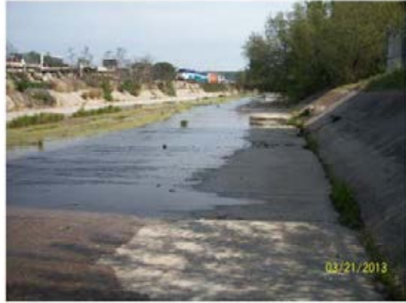
58. Reach 3 - Looking south from within the channel from a point approximately 920 feet south of the Sorrento Valley Blvd bridge.
