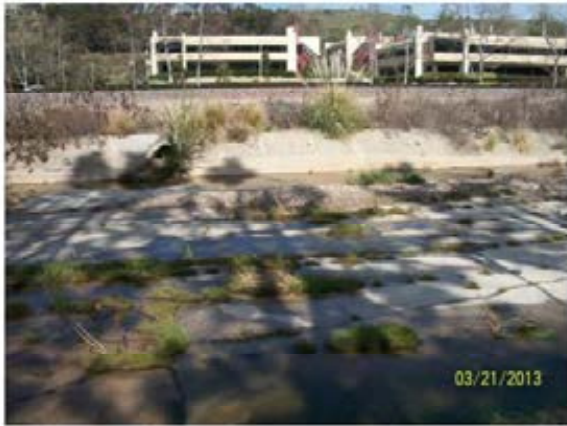
59. Reach 3 – Looking east at sediment deposition located at the upstream end of Reach 3.
