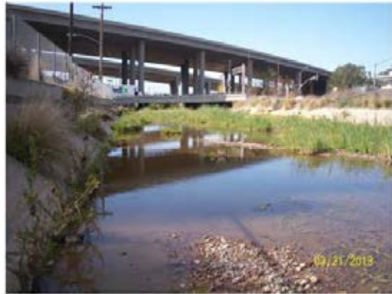
46. Reach 3 - Looking north at the upstream side of the Sorrento Valley Blvd bridge from within the west side of the channel.
