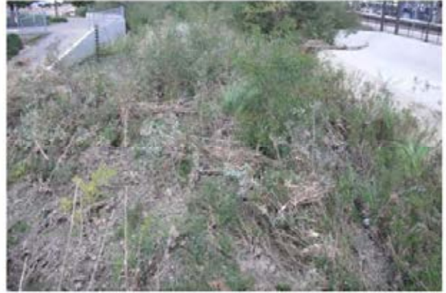
34. Reach 3 – Looking north from the top of the pedestrian bridge that crosses Reach 3 near its downstream end.
