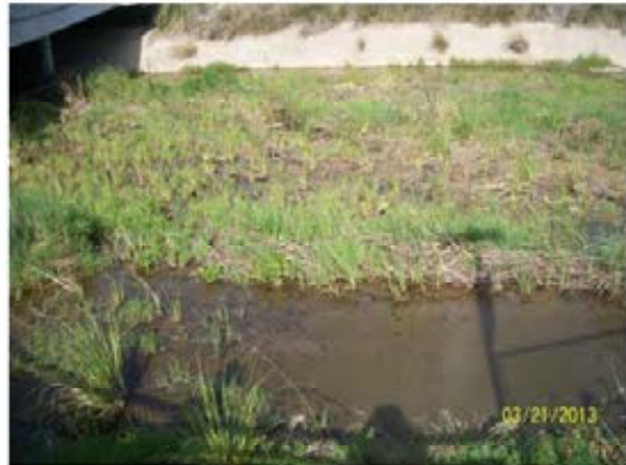
44. Reach 3 – Looking east just upstream of the Sorrento Valley Blvd bridge from Roselle Street.
