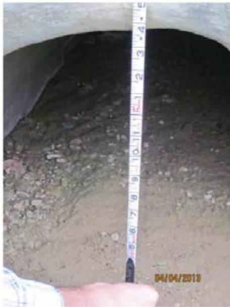
63. Reach 7 – Close up view of the measuring tape over the 30-inch RCP. The measuring tape shows that the sediment deposition depth at this location is 14-inches ( 30'' - 16'' = 14'' ).
