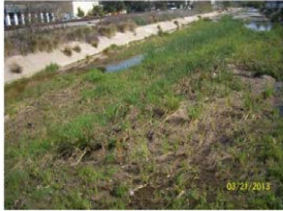
42. Reach 3 – Looking southeast from the top of the Sorrento Valley Blvd bridge.
