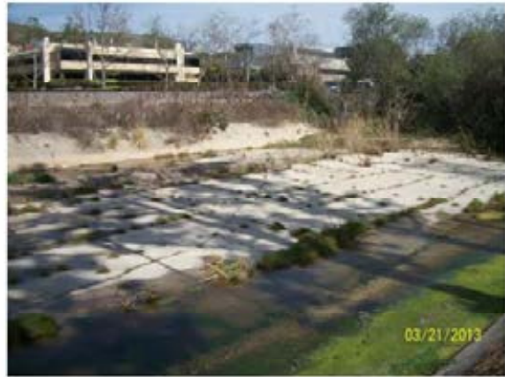
60. Reach 3 – Looking southeast at sediment deposition located at the upstream end of Reach 3.
