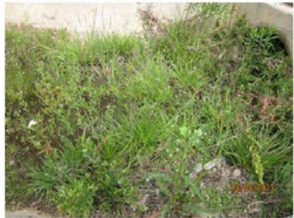
80. Reach 7 – Looking at the dual 36-inch RCP culvert entrance that discharges into the Sorrento Creek Channel. The vegetation, sediment deposition, and other debris are visible.
