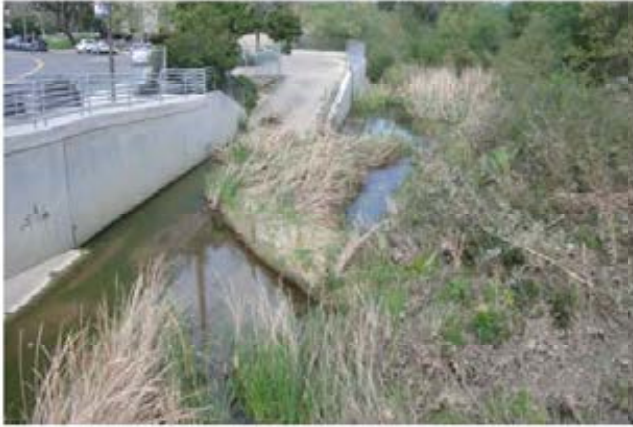
33. Reach 3 – Looking north from the top of the pedestrian bridge that crosses Reach 3 near its downstream end.
