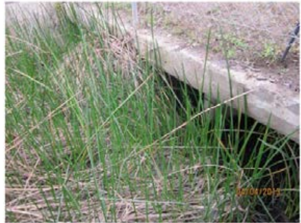
74. Reach 7 – Close up view of the Roselle Street culvert entrance (west side). The high vegetation density blocking the entrance of the culvert and ponded water within the culvert are visible this photo.
