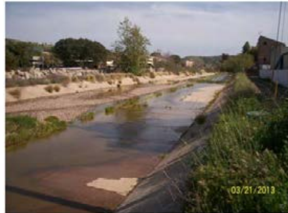
56. Reach 3 - Looking south from the west side channel bank near Roselle Street and approximately 600 feet to the southeast of the Sorrento Valley Blvd bridge.
