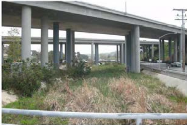
37. Reach 3 – Looking south from the top the of pedestrian bridge that crosses Reach 3 near its downstream end.
