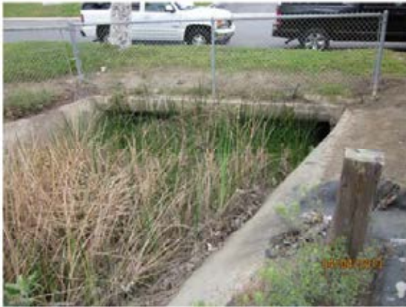
73. Reach 7 – Looking east at the upstream (west) side of the Roselle Street culvert. The high density of the vegetation blocking nearly 40% to 50% of the cross sectional area of the culvert can be appreciated in this photo.
