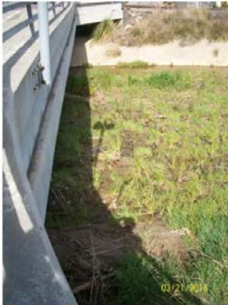
43. Reach 3 – Looking east at the upstream side of the Sorrento Valley Blvd bridge from the top of the bridge.
