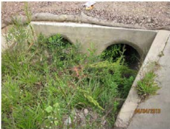
79. Reach 7 – Looking at the dual 36-inch RCP culvert entrance that discharges into the Sorrento Creek Channel. The vegetation, sediment deposition, and other debris are visible.
