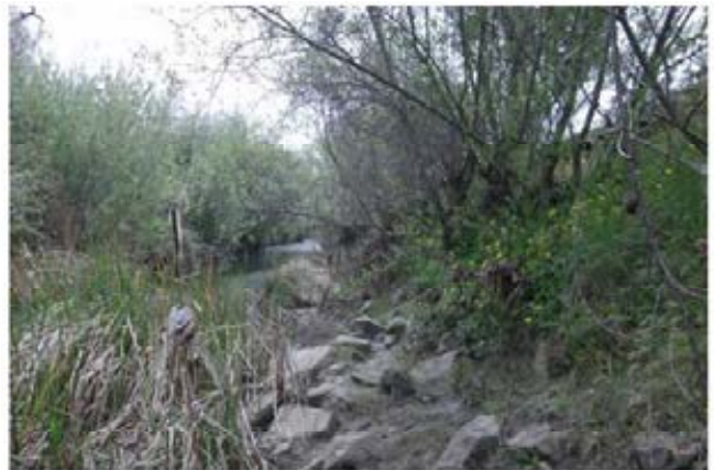
20. Reach 2 – Vegetation growth through riprap along the west bank.
