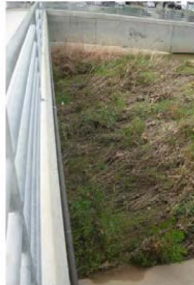
36. Reach 3 – Looking at the downstream side of the Reach 3 pedestrian bridge in a westerly direction.
