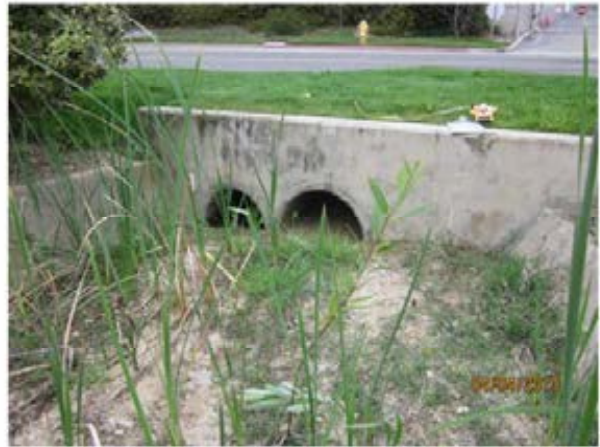
62. Reach 7 - Looking west at the upstream end of Reach 7 where it receives the flow from a 24-inch and a 30-inch RCP.
