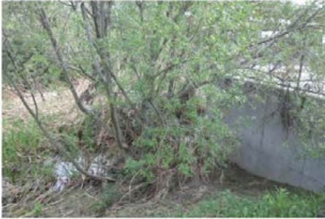
25. Reach 2 - Looking south at the north end of the reach, where Reach 2 begins to widen as it transitions to the concrete-lined channel Reach 3.
