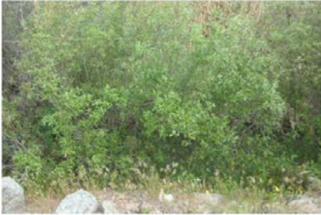
17. Reach 2 – Dense vegetation growth through riprap along the west bank.
