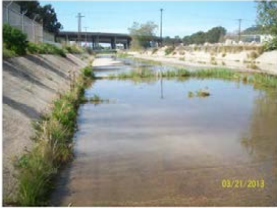
57. Reach 3 - Looking north from within the channel from a point approximately 920 feet south of the Sorrento Valley Blvd bridge.
