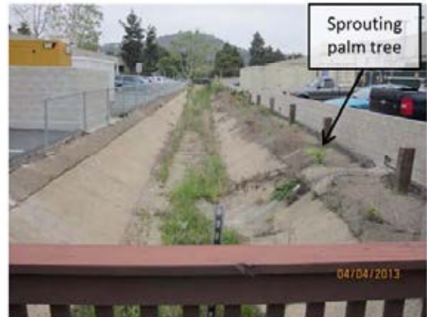
70. Reach 7 – Looking east from the wooden pedestrian bridge that is located approximately 400 feet east of Flintkote Avenue. There is very little to no sediment deposition downstream from the bridge; however, there is minimal vegetation growth, which if left unchecked could encourage more sediment deposition. This photo also shows a sprouting palm tree on the south bank, which could potentially damage the structural integrity of the concrete channel in the future.
