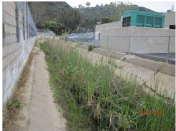
68. Reach 7 – Looking west in an upstream direction. The sediment deposition along this section of the reach is approximately 4 to 6 inches.
