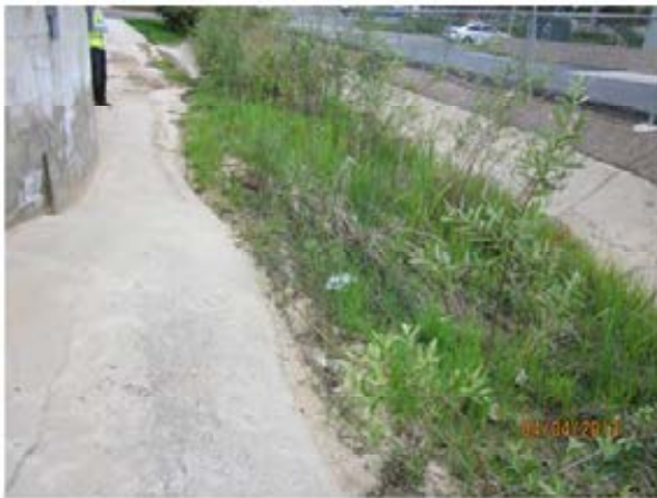
67. Reach 7 – Looking west in an upstream direction. The sediment deposition along this section of the reach is approximately 4 to 6 inches.
