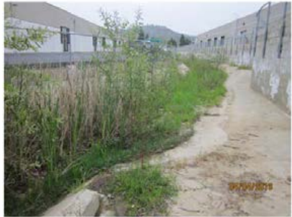
66. Reach 7 - Looking east in a downstream direction from the channel access ramp.
