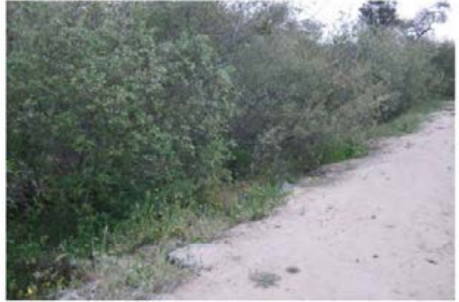
18. Reach 2 – Dense vegetation growth through riprap along the west bank.
