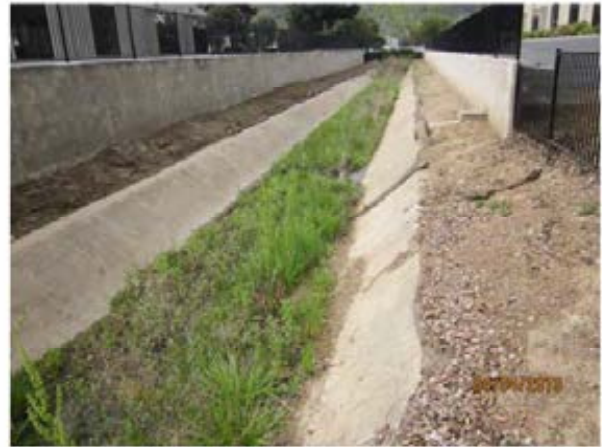
78. Reach 7 – Looking in an upstream direction from the downstream end.
