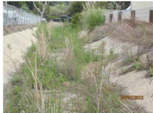
72. Reach 7 – Looking east in downstream direction. Although along this section of the reach, sediment is approximately 0 to 0.5 inch deep, the vegetation starts to get denser starting at a location 170 feet upstream from the Roselle Street culvert.
