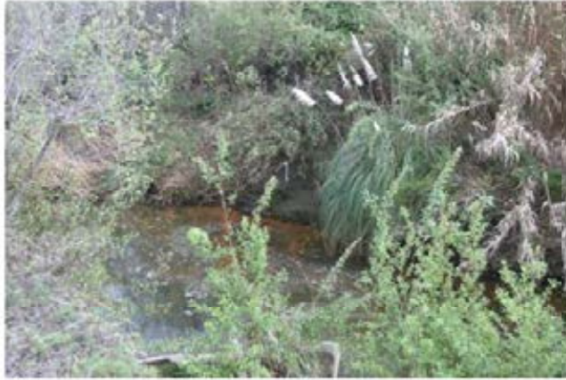
21. Reach 2 – Looking east, the Dunhill Street 54-inch RCP headwall is visible at the lower side of the photo. Notice the narrow channel top width.
