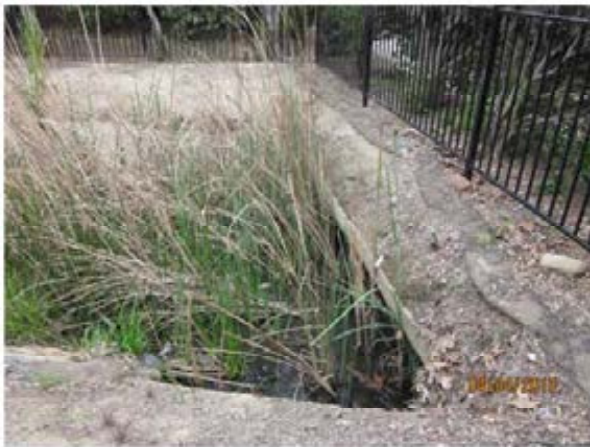
75. Reach 7 – Looking south at the outlet of the Roselle Street culvert. Vegetation, sediment deposition, debris, and ponded water are visible.
