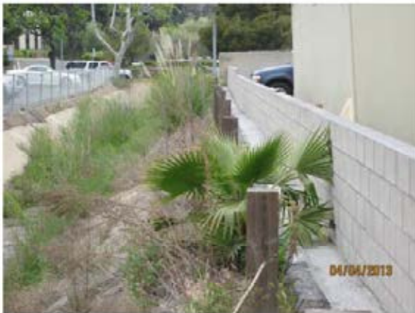
71. Reach 7 – Looking east in a downstream direction along the south bank. At a location approximately 100 feet from the wooden pedestrian bridge, a juvenile palm tree is visible in this photo on the south bank, which could potentially damage the structural integrity of the concrete channel in the near future.
