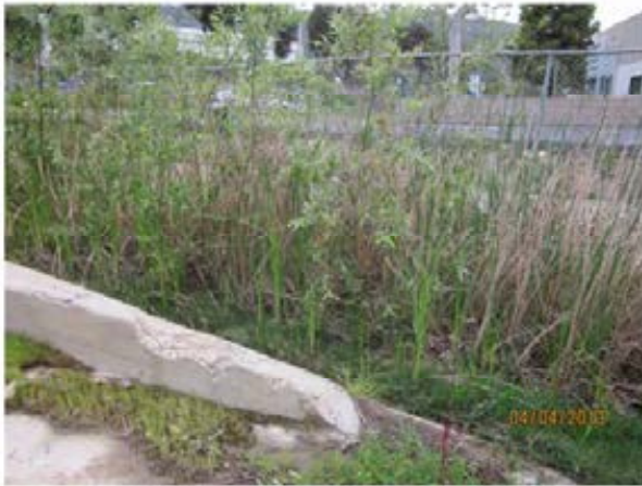
65. Reach 7 – Looking north across Reach 7, near the upstream end from the channel access ramp.
