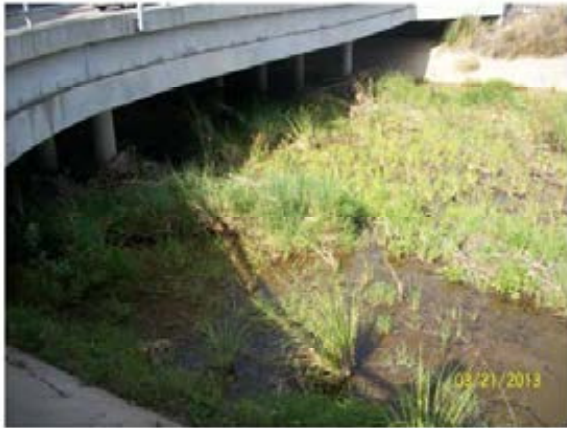
45. Reach 3 – Looking northeast at the upstream side of the Sorrento Valley Blvd bridge.
