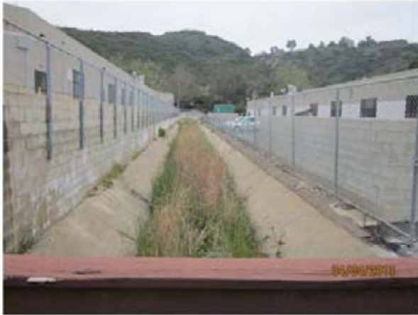
69. Reach 7 – Looking west from the wooden pedestrian bridge that is located approximately 400 feet east of Flintkote Avenue. The sediment deposition decreases in a downstream direction, and it disappears at the bridge.
