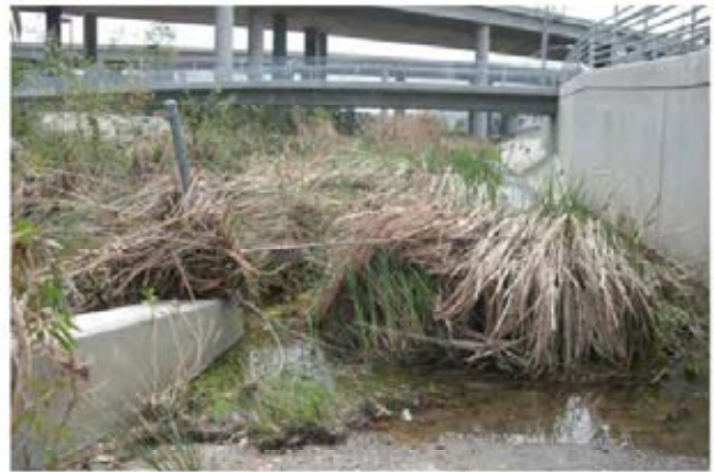
32. Reach 3 – Looking south from the channel access ramp located at the downstream end of Reach 3, close up view.
