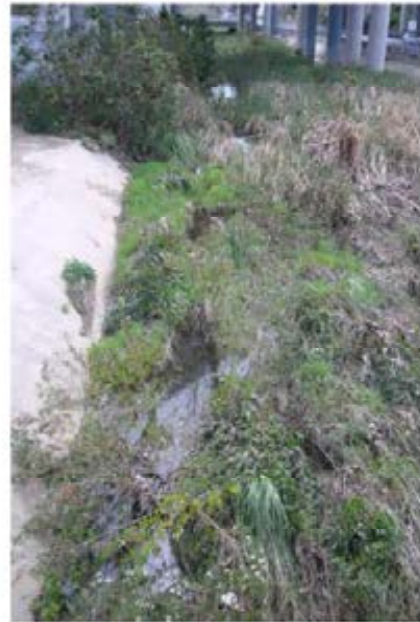
38. Reach 3 – Looking south from the top the of pedestrian bridge that crosses Reach 3 near its downstream end.
