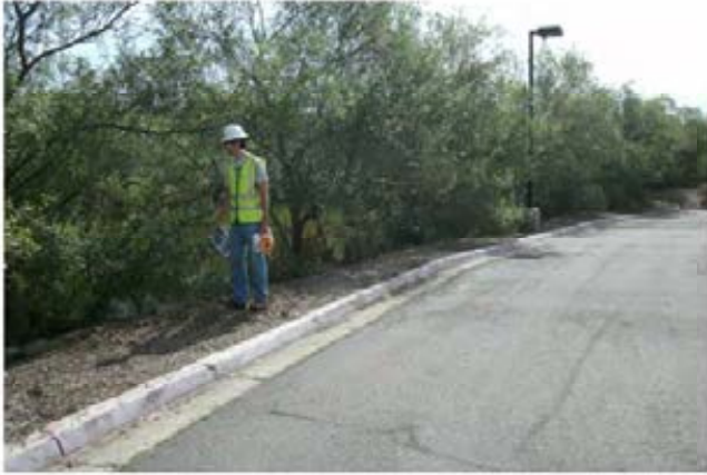
5. Reach 1 – Light to dense vegetation is visible along the westerly bank of Reaches 1 and 2. Although not completely visible in this photo, riprap is barely visible at the lower left corner of this photo.
