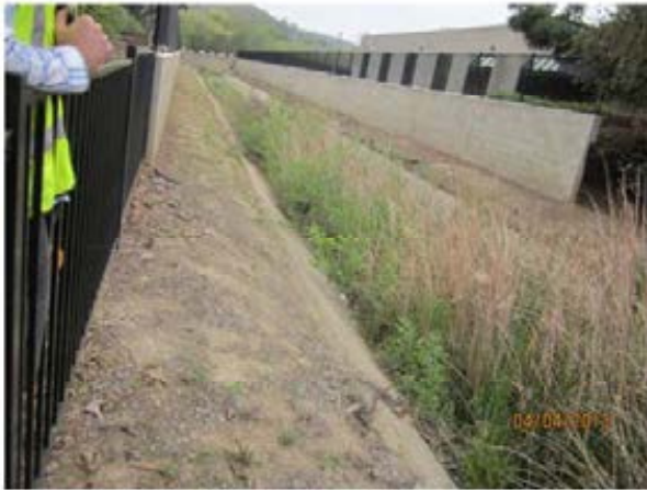
77. Reach 7 – Looking east in a downstream direction. Most of Reach 7, downstream from Roselle Street is visible.
