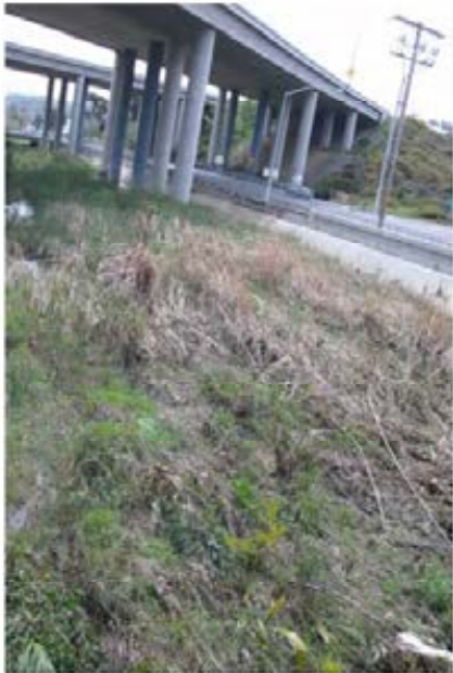
39. Reach 3 – Looking southwest from the top of the pedestrian bridge that crosses Reach 3 near its downstream end.
