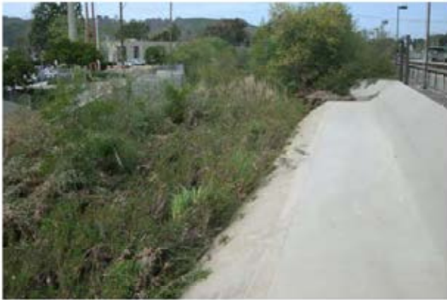
35. Reach 3 – Looking north from the top of the pedestrian bridge that crosses Reach 3 near its downstream end.
