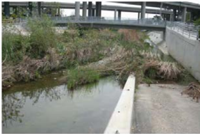
31. Reach 3 – Looking south from the channel access ramp located at the downstream end of Reach 3.
