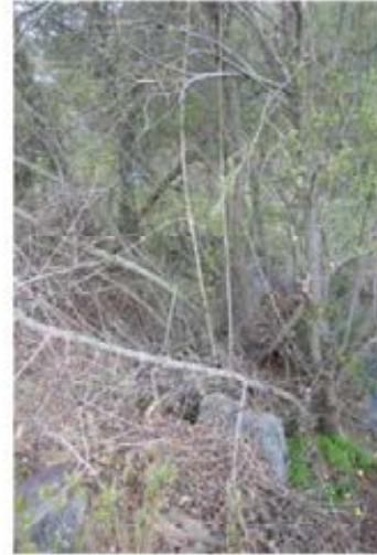
6. Reach 1 – Vegetation is visible along the westerly bank growing through the riprap, typical of Reaches 1 and 2.
