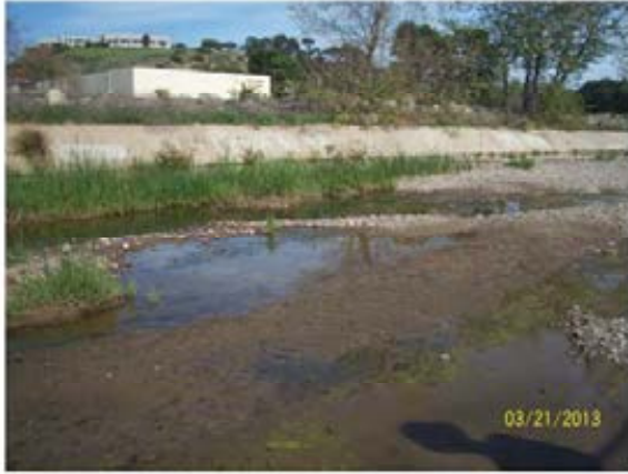
49. Reach 3 - Looking southeast from within the west side of the channel bed at point approximately 450 feet south of the Sorrento Valley Blvd bridge.
