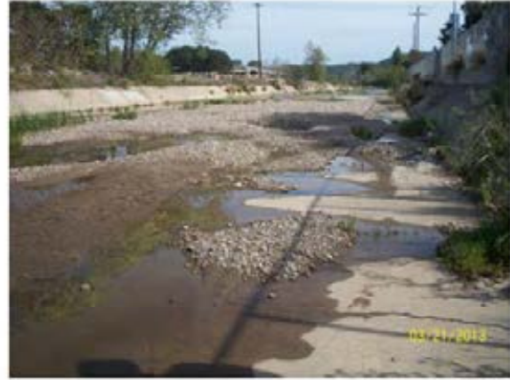
50. Reach 3 - Looking southeast from within the west side of the channel bed at point approximately 450 feet south of the Sorrento Valley Blvd bridge.
