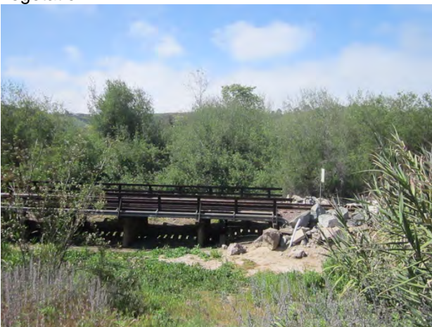
Photo #25 View: SW Historic resource CA-SDI-16385 – Former Atchison-Topeka & Santa Fe Railroad
