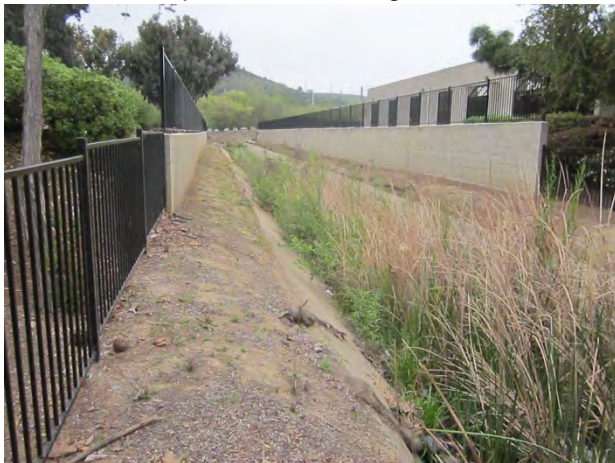
Photo #: 9 View: SW Canal adjacent to Reach 7 Access - Cement lined with constructed 2-foot walkway on either side
