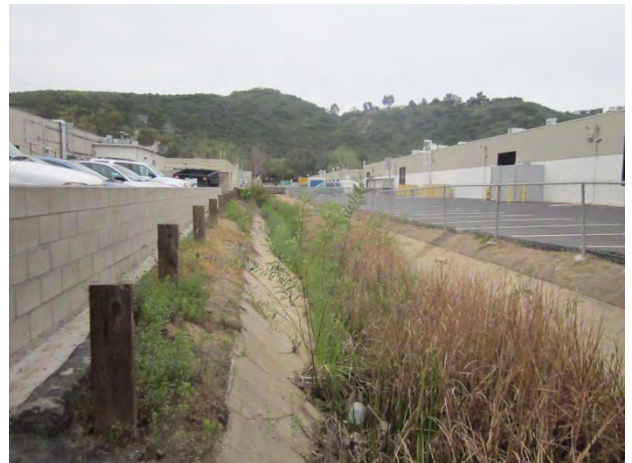
Photo #:10 View: SW Reach 7 - 100 percent cement-lined
