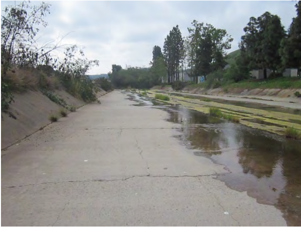
Photo #: 17 View: SE Reach 3 - East of Interstate Highway 5
