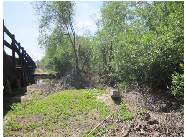
Photo #: 23 View: SE At rail bridge, north bank of Reach 1 blocked by vegetation
