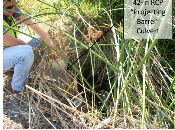
18. PBO downstream end at 42-inch culvert. High vegetation density observed at the entrance to the 42-inch projecting barrel (no headwall) type culvert where the earthen channel discharges. The vegetation obstructs approximately 50 percent of the cross sectional area of the 42-inch drainpipe.
