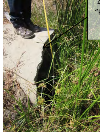
36. PBO downstream end at 42-inch culvert. Denser vegetation is observed than the previous year at the entrance of the culvert; however, sediment deposition and ponded water depth are approximately the same.
