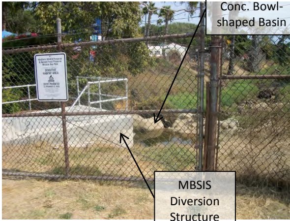
21. Outfall at Pacific Beach Drive/Olney Street intersection. The MBSIS diversion structure is located at the downstream end of the 42-inch culvert. Water is ponded at the exit of the structure in a concrete bowl-shaped basin.
