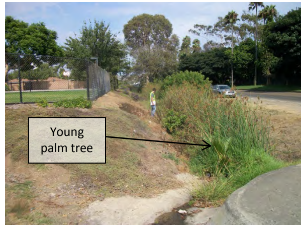
20. PBO - At Olney Street looking east. It was observed that vegetation on the north side slope is very light. Additionally, a young palm tree is growing adjacent to the culvert entrance, which in the near future could damage the entrance to the culvert and further reduce the capacity of the culvert.
