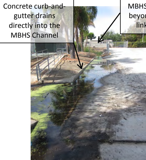
25. MBHS – Dry-weather non-storm water backing up the concrete channel and into the school bus loading\unloading zone of Mission Bay High School. Notice how the removal of the vegetation at the outlet of the 27-inch RCP does not remediate the flooding in this area.
