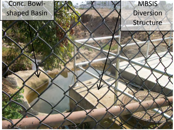
22. Outfall at Pacific Beach Drive/Olney Street intersection. This image shows another view of MBSIS concrete diversion structure and concrete bowl-shaped basin.
