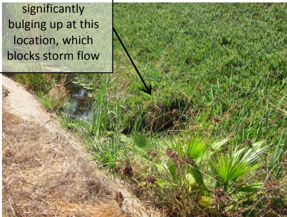
29. MBHS – North edge of southerly parking lot looking south. Dry weather ponded water is observed at about the same depth as previous year. The ice plant has completely covered the west side of the channel and has partially grown across the concrete channel bottom. Notice that as a result of a denser ice plant, it is actually bulging up.
