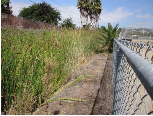
27. MBHS – South of Baseball field looking north. Existing vegetation is ~6 ft., within the concrete channel, approximately of the same height along this section of the channel, but denser than previous year.
