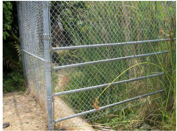
10. MBHS – South end at edge of high school. High amounts of trash and vegetation growth were observed within the channel. Vegetation growth could become an obstruction to storm flow during a major storm event.
