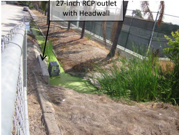
23. MBHS - Upstream end – 27-inch RCP outlet with Headwall. Existing vegetation that was obstructing the outlet of the existing 27-inch RCP has been removed in an effort to minimize flooding impacts and back flows.
