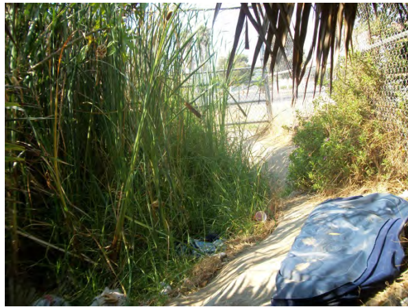
11. MBHS – Downstream end/Pacific Beach DR/Olney upstream end. Transition of concrete channel to earthen channel. Large amounts of vegetation growth and debris were observed.
