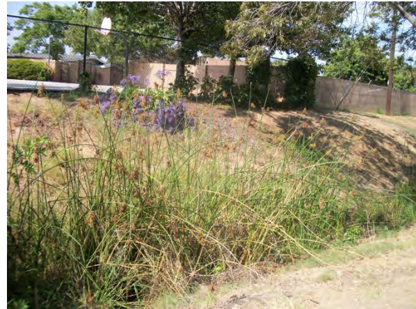
16. PBO - approximately 200 feet upstream of 42-inch culvert sections where vegetation tends to be lighter were observed. This image illustrates one of two sections where the vegetation growth was lighter.
