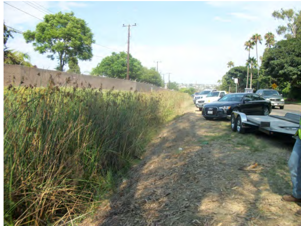
15. PBO - approximately midpoint of channel looking east. The high vegetation density and growth on the channel bed, and light vegetation growth on the south channel side slope is representative of the conditions along the earthen channel.
