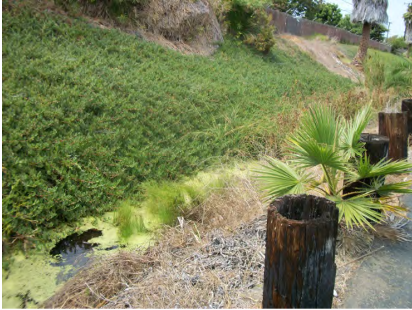
7. MBHS – North edge of southerly parking lot looking north. Dry weather ponded water is observed. The ice plant has completely covered the west side of the channel and has partially grown across the concrete channel bottom.
