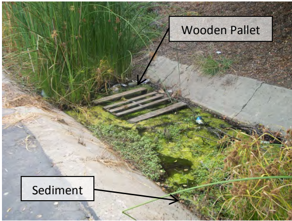
9. MBHS – Midpoint of southerly parking lot. The 3 to 4-inch thick sediment layer was observed, as well as the ponded water, trash, and even a wooden pallet within the channel. The concrete channel is visible in this area.
