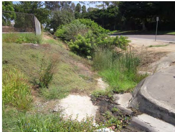
37. PBO - At Olney Street looking east. It was observed that vegetation at approximately 25 feet from the culvert is denser than the previous year. A young palm tree that was growing very close to the culvert the previous year seems to have been removed as it was not visible during the last site visit.
