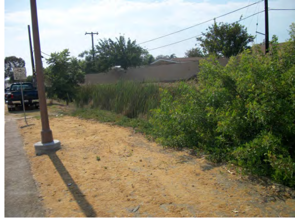
14. PBO - upstream end looking west. High vegetation density observed.
