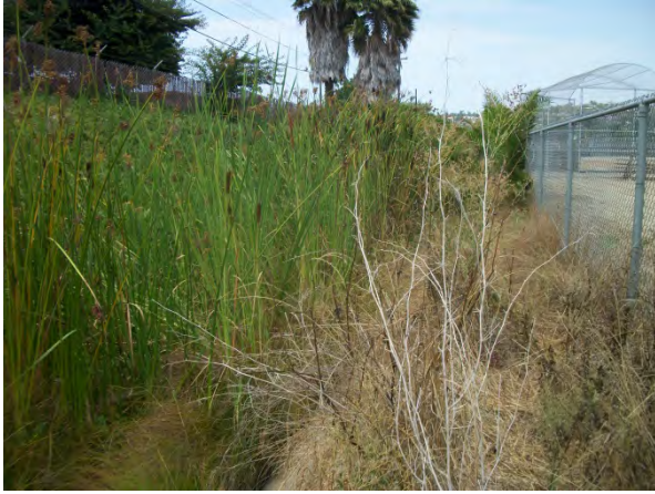
5. MBHS – South of Baseball field looking north. Existing vegetation is ~6 ft., within the concrete channel.
