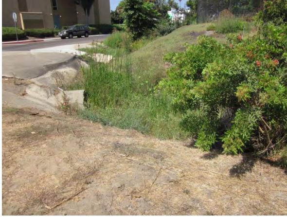
35. PBO - downstream end looking east. The denser vegetation growth than the previous year is observed.
