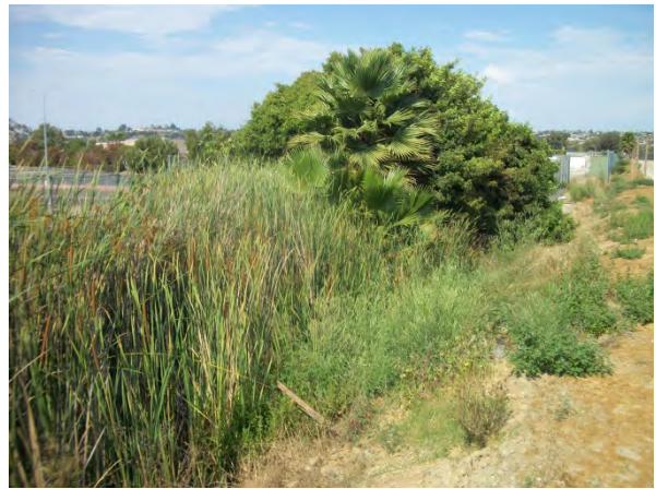
12. PBO - upstream end looking east. High vegetation density and growth were observed at the upstream end of the earthen channel.
