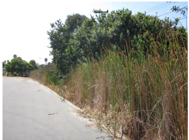
30. MBHS – North edge of southerly parking lot looking south. Existing vegetation is ~8-10 ft. high, within the concrete channel, denser and taller than previous year.
