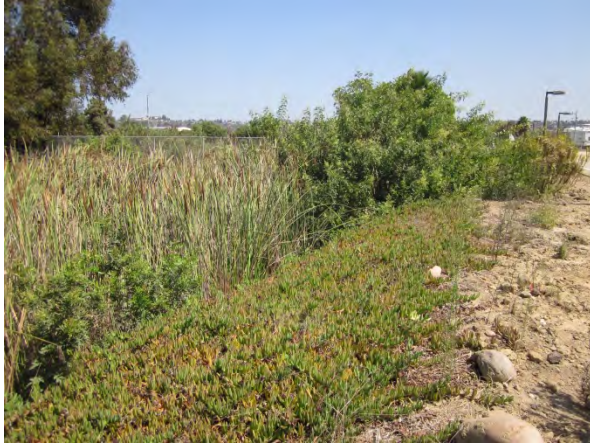
31. PBO - upstream end. Taller and denser vegetation growth than previous year at the upstream end of the channel.
