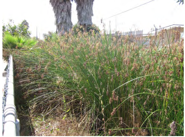
28. MBHS – South of Baseball field looking south. Existing vegetation is ~8 ft., within the concrete channel, taller and denser along this section of the channel than previous year.
