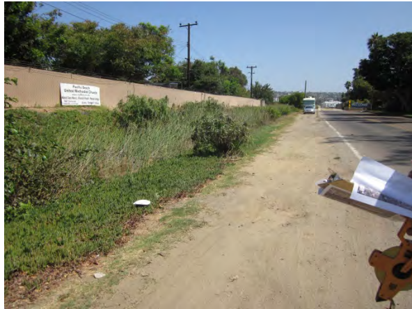
33. PBO - approximately midpoint of channel looking east. The denser vegetation growth on the channel bed than previous year, and similar vegetation growth on the south channel side slope are visible.
