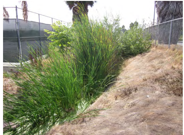
24. MBHS - Downstream of headwall. Notice that the amount of growth and density of the existing vegetation within the MBHS concrete channel is significantly denser than the previous year.
