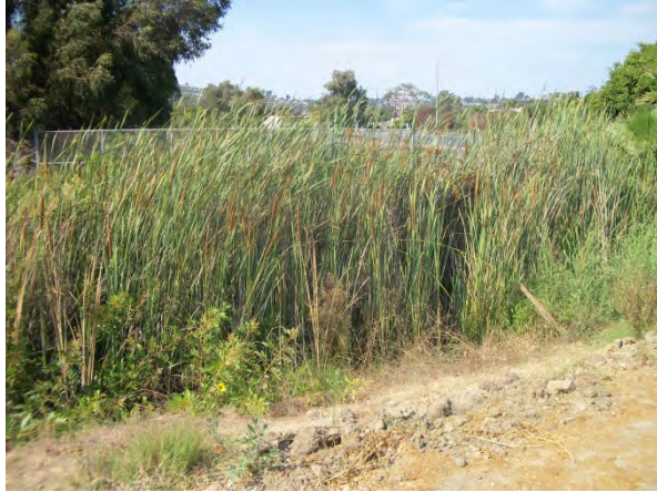
13. PBO - upstream end. High vegetation density and growth at the upstream end of the earthen channel were observed.
