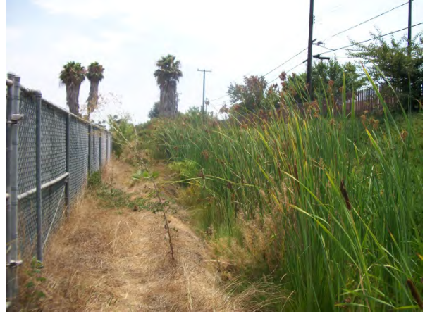
6. MBHS – South of Baseball field looking south. Existing vegetation is ~6 ft., within the concrete channel.
