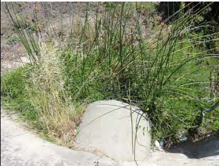
Culvert located at downstream end of Pacific Beach/Olney Street Channel. No standing or flowing water observed
