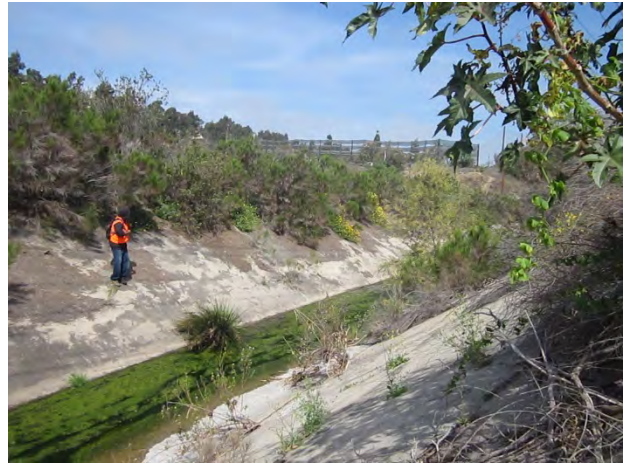
Photo #: 45 View: NW Channel 58a – Cement-lined from bank to bank
