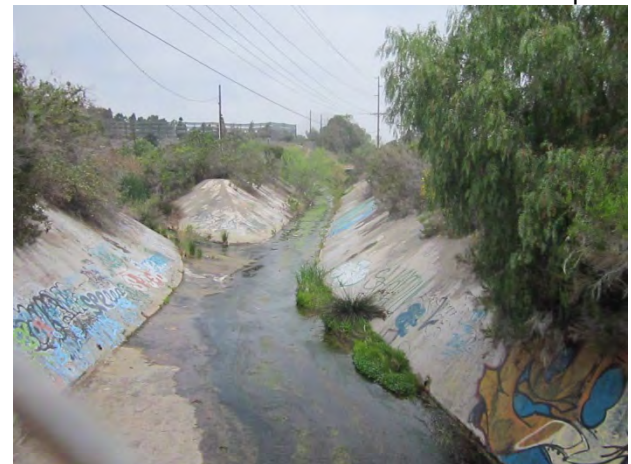
Photo #: 43 View: N Cement lined convergence of Channel 58a & 58b
