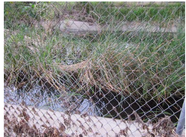
Photo #: 41 View: E Channel 58 - Cement lined with sediments and plants
