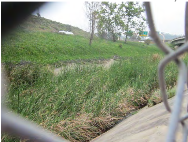
Photo #: 42 View: N Channel 58 – Overview of cement-lined northern segment
