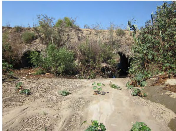
24. SG Channel – Triple 72-inch CMPs entrance (upstream) at Disney Crossing. The middle pipe entrance is almost completely covered with vegetation, sediment deposition, trash and debris. The high levels of sediment deposition is visible immediately upstream of the entrance.
