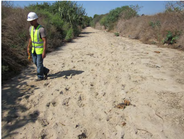
23. SG Channel – Looking north (upstream) from a point approximately 50 feet downstream from the Disney Crossing. The high amount of sediment deposition is visible on the streambed.
