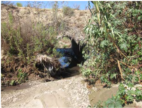
72-inch CMP outlet covered with vegetation
