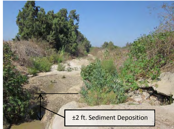
16. SG Channel – Looking north near the outlet of the 52-inch CMP culvert under Monument Road.
