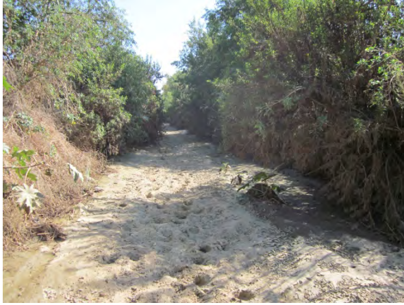
29. SG Channel – Looking south (upstream) at a point approximately \pm 450 feet upstream of the Pilot\SG channel confluence. The high amount of sediment deposition is visible on the streambed.
