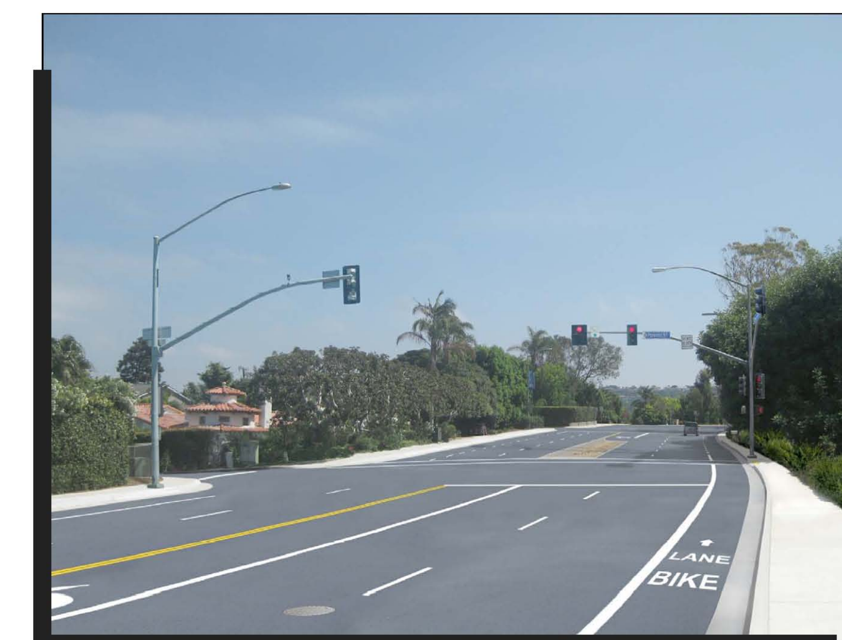
KEY VIEW 4 - LOCATION EVALUATED FOR TRAFFIC SIGNAL AT TORREY PINES RD. & PRINCESS ST.
