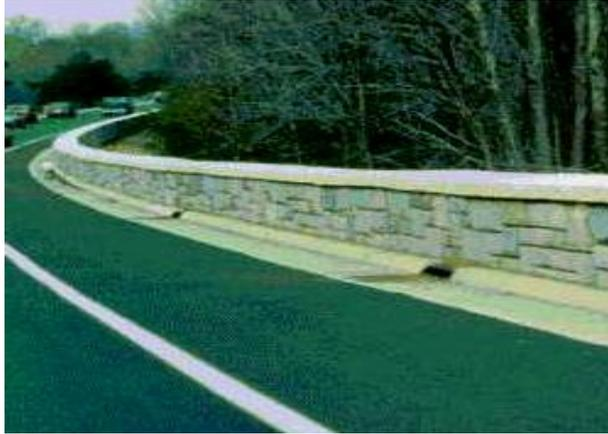
A Precast Concrete Guardwall Installation
