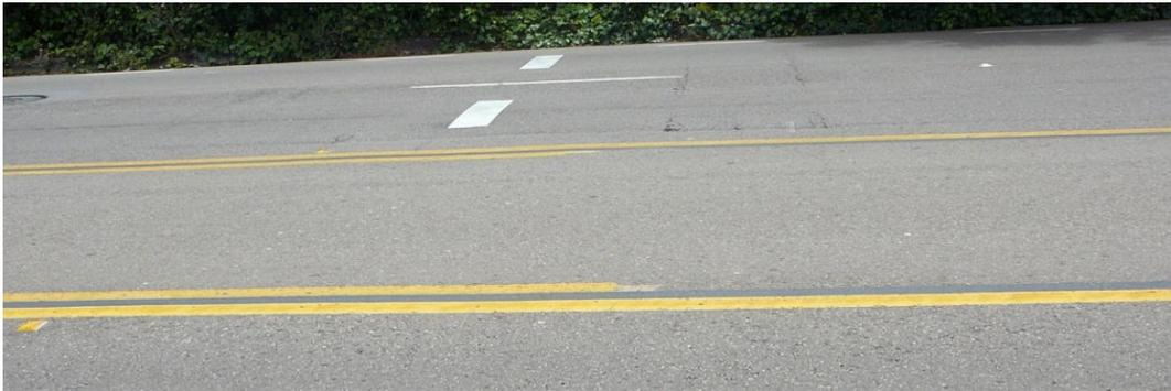
Picture 3965 - Solid Yellow and Broken Yellow Stripes on Each Side of Median
