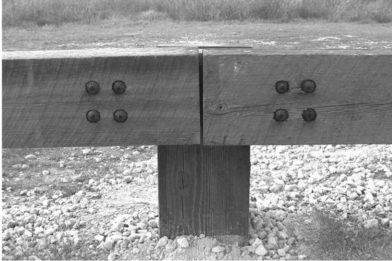
Timber Guardrail Post Detail
