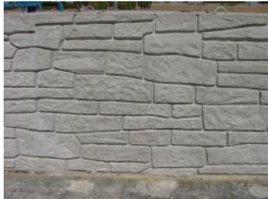
Type 60 Concrete Barrier with aesthetic treatment
