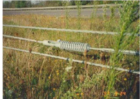
Three-Cable barrier installed in Oregon.
