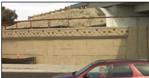
*Concrete Retaining wall, soil nail and shotcrete support along Interstate 5*
