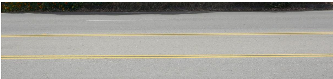
Picture 3966 - Double Solid Yellow Strips on Each Side of Median
