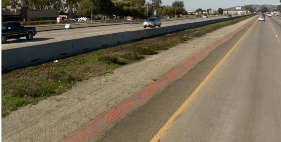
Grooved Pavement on freeway (also note decorative strip at edge of shoulder)
