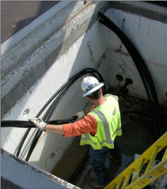
Crew member installs new underground cables.
