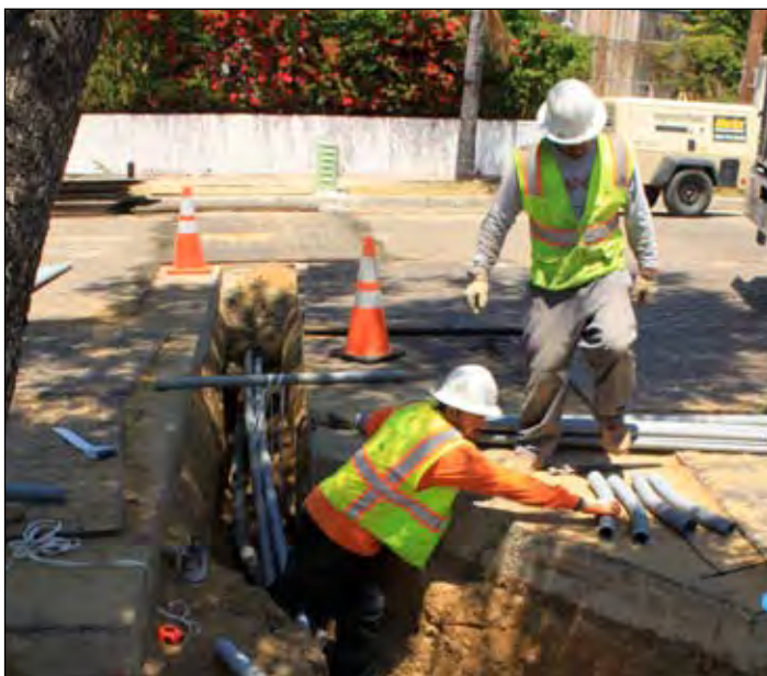
Construction crew members place new underground conduits in open trench.
