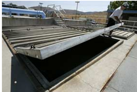
RONI GALGANO / Union-Tribune Don Denniston lifted a cover over sewage that is pumped into a recycling plant at the Padre Dam water district.
