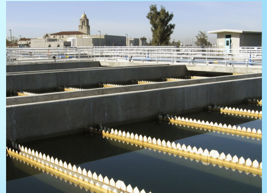
Alvarado Water Treatment Plant, one of San Diego's drinking water treatment facilities
