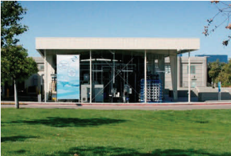
Advanced Water Purification Facility
