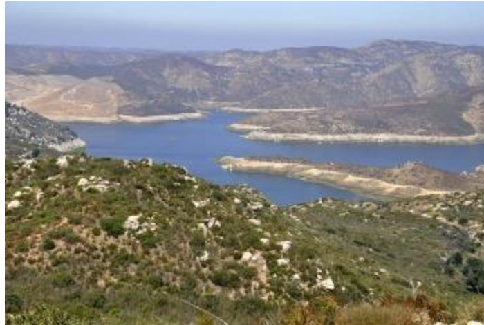
San Vicente Reservoir, August 2010. Water level has been lowered to allow dam raise construction.
