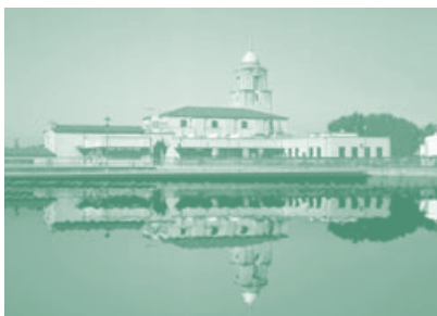
Alvarado Water Treatment Plant
