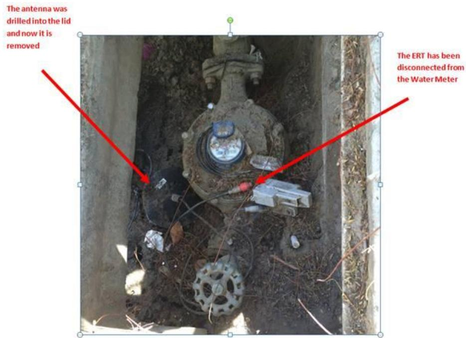
You are responsible when working in and around meter boxes. If you encounter these endpoints, use proper care and do not disconnect them from the registers on top of the water meter. Also if the lid has an antenna drilled through, do not change or tamper with the lid and inform the Resident Engineer about the location of that lid.
