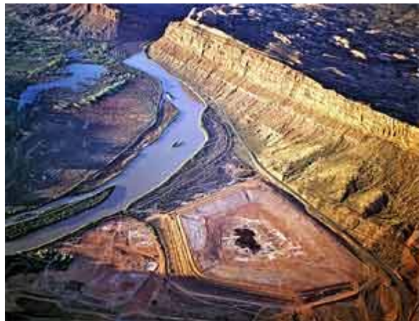
Associated Press An aerial photograph shows the pile of radioactive waste along the Colorado River in Moab, Utah, that will be moved to another Utah site about 30 miles from the river.
