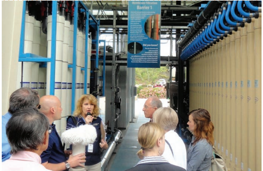
Members of the public receive a free tour of the City of San Diego's Advanced Water Treatment Facility as part of the Water Purification Demonstration Project.
