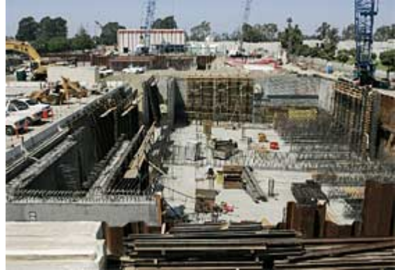
CHARLIE NEUMAN / Union-Tribune Starting in 2007, the Orange County Water District's Fountain Valley plant is expected to provide enough drinking water for the equivalent of 140,000 families.
