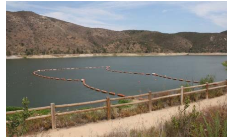
Figure 4-5. Emergency Pump Storage Area, Site 4
