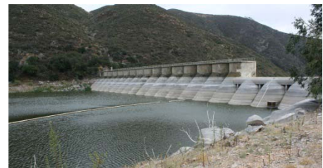
Figure 4-2. Lake Hodges Dam Area, Site 1
