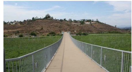
Figure 4-6. Lake Hodges Pedestrian Bridge, Site 6
