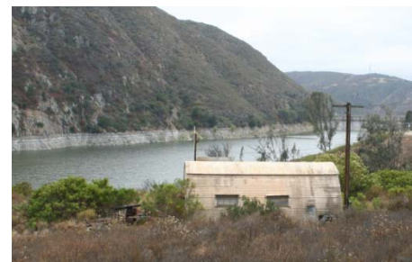
Figure 4-3. Former Reservoir Operator Residence and Storage Facility Area, Site 2
