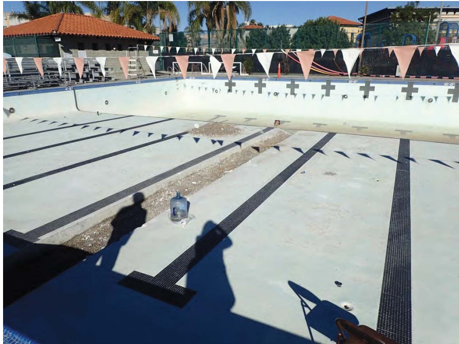
Photograph 1: Drained pool with sawcut area, view to northwest. 12/19/18
