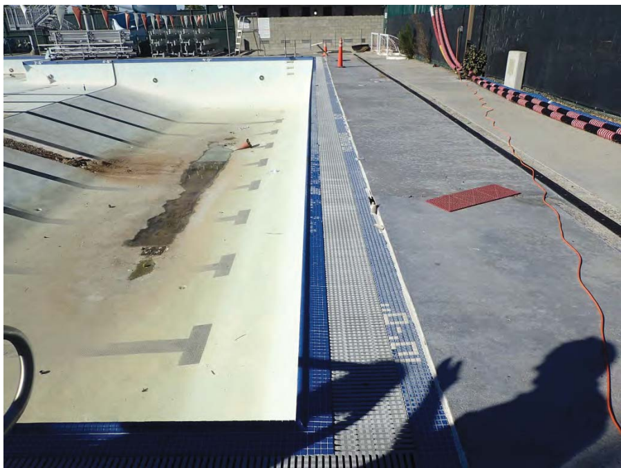
Photograph 2: North side of pool, view to west. Pool wall exhibits bowing. 12/19/18
