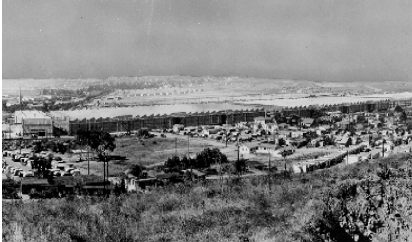
Consolidated Aircraft, 1940s, looking southwest.
