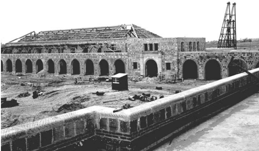
The Marine Corps Recruit Depot under construction.
