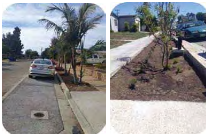
Figure 4-8 Bannock Avenue During Construction
