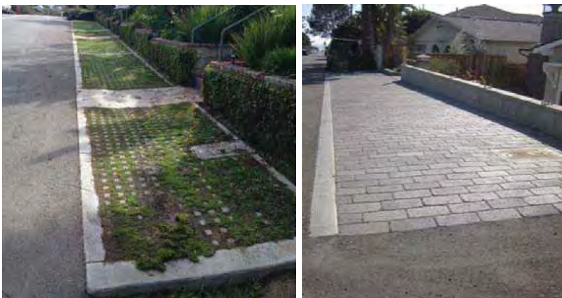
Figure 4-7 Permeable Pavers in the Right-of-Way Without Curb and Gutter
