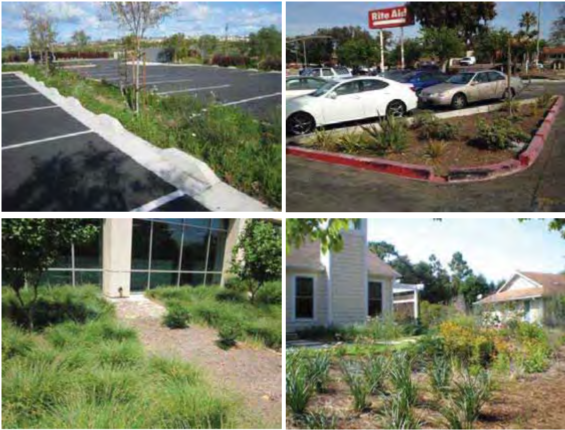
Figure 4-4 Bioretention Areas in Parking Lots and Adjacent to Buildings Provide Multiple Benefits by Treating Runoff While Also Serving as Landscape Features and Habitat
