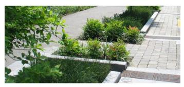
Green infrastructure can help filter storm water before it enters the conveyance system.
