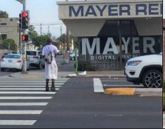
Advance Stop Bars/Limit Lines direct drivers where to stop at intersections and mid-block crossing locations, providing separation between the vehicle and crossing pedestrians.
