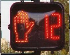
**Pedestrian Countdown Signals** provide pedestrians with a clear indication of how many seconds remain to safely cross.
