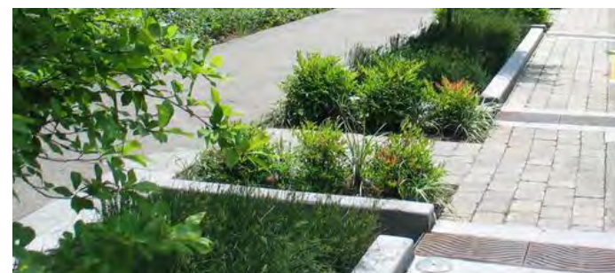
Green infrastructure can help filter storm water before it enters the conveyance system.
