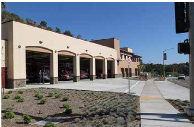
Station 45 provides fire and rescue services to the eastern area of Mission Valley.
