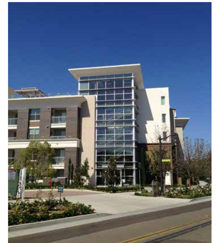
Adequate access to natural light can minimize energy costs.
