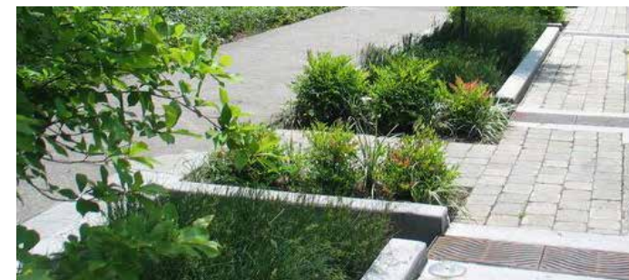
Green infrastructure can help filter storm water before it enters the conveyance system.
