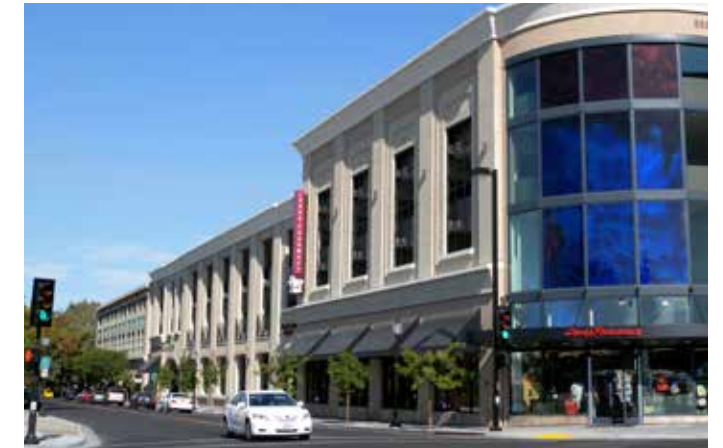
The structured parking (above ground floor) is designed as an integral part of the building through consistent architectural style and materials.
