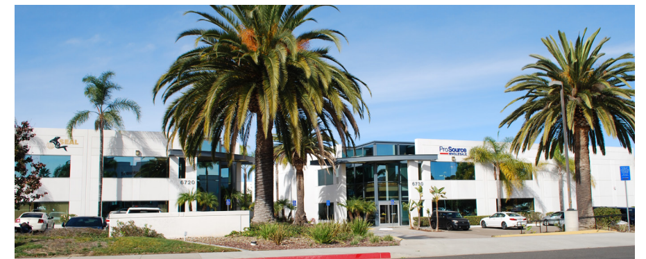
Office complex on Top Gun Street
