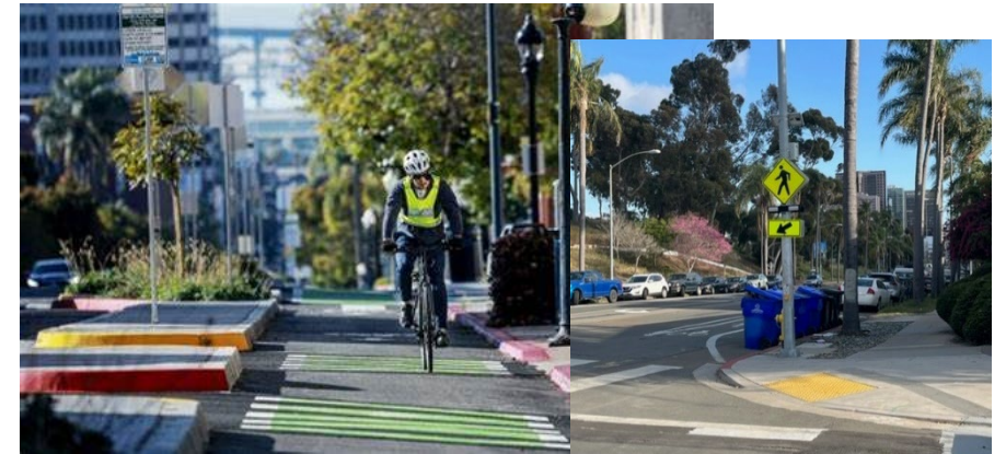
Enhanced pedestrian crossings and separated bike lane on 4 th and 5 th Avenue
