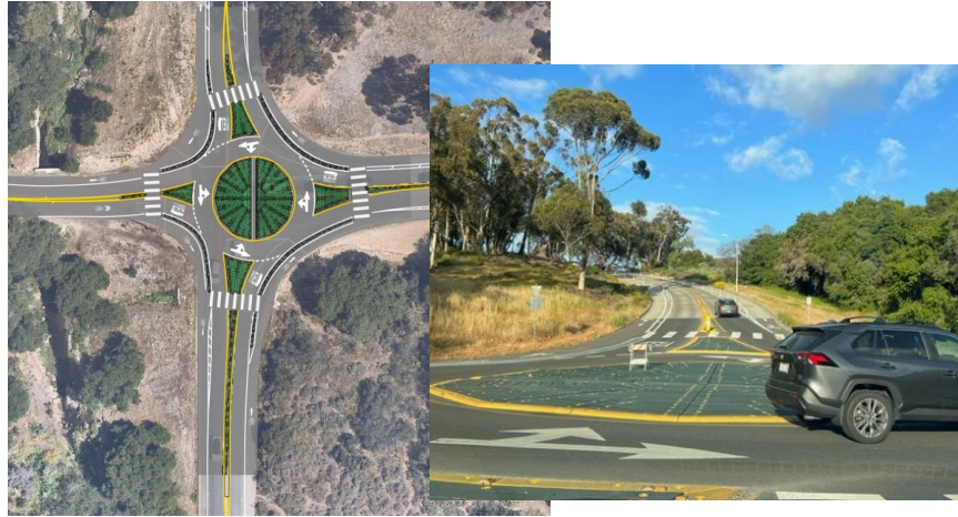
Quick-build roundabout on Florida Drive
