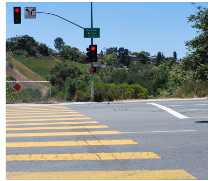
5. Advanced Stop Bars/Limit Lines direct drivers where to stop at intersections and mid-block crossing locations, providing separation between the vehicle and crossing pedestrians.
