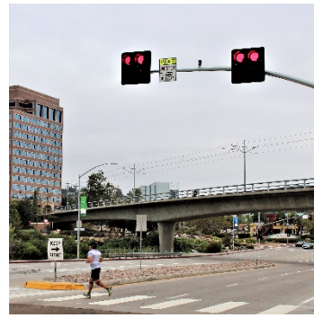
6. Pedestrian Hybrid Beacons are traffic control signals that help pedestrians and bicyclists cross mid-block across high traffic roadways.
