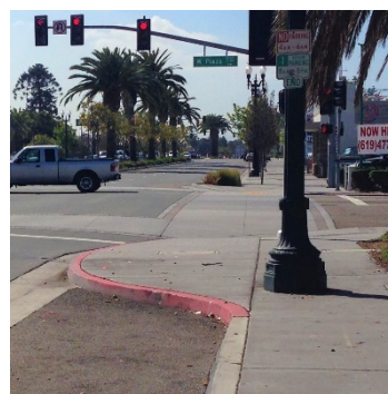
3. Curb Pop Outs or Curb Extensions shorten pedestrian crossing distances and serve as a traffic calming mechanism.
